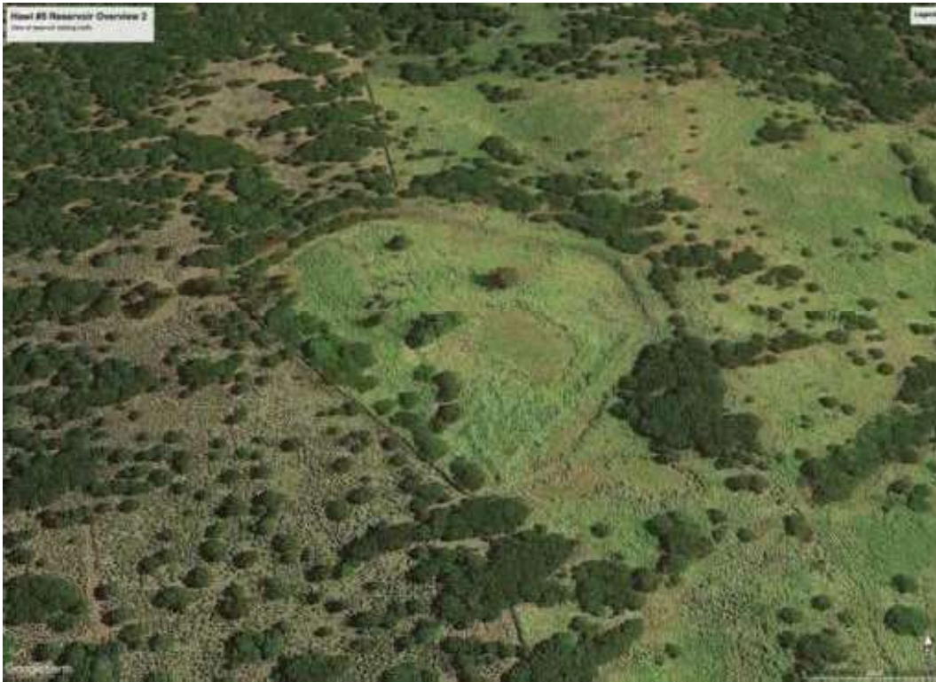
Figure 4. Hawi No. 5 reservoir basin.
