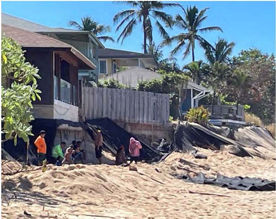
Figure 2 Work crews on October 28, 2023
