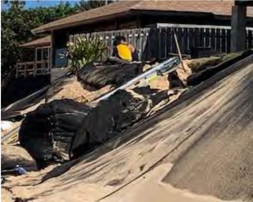
Figure 3 Work crews on November 4, 2023
