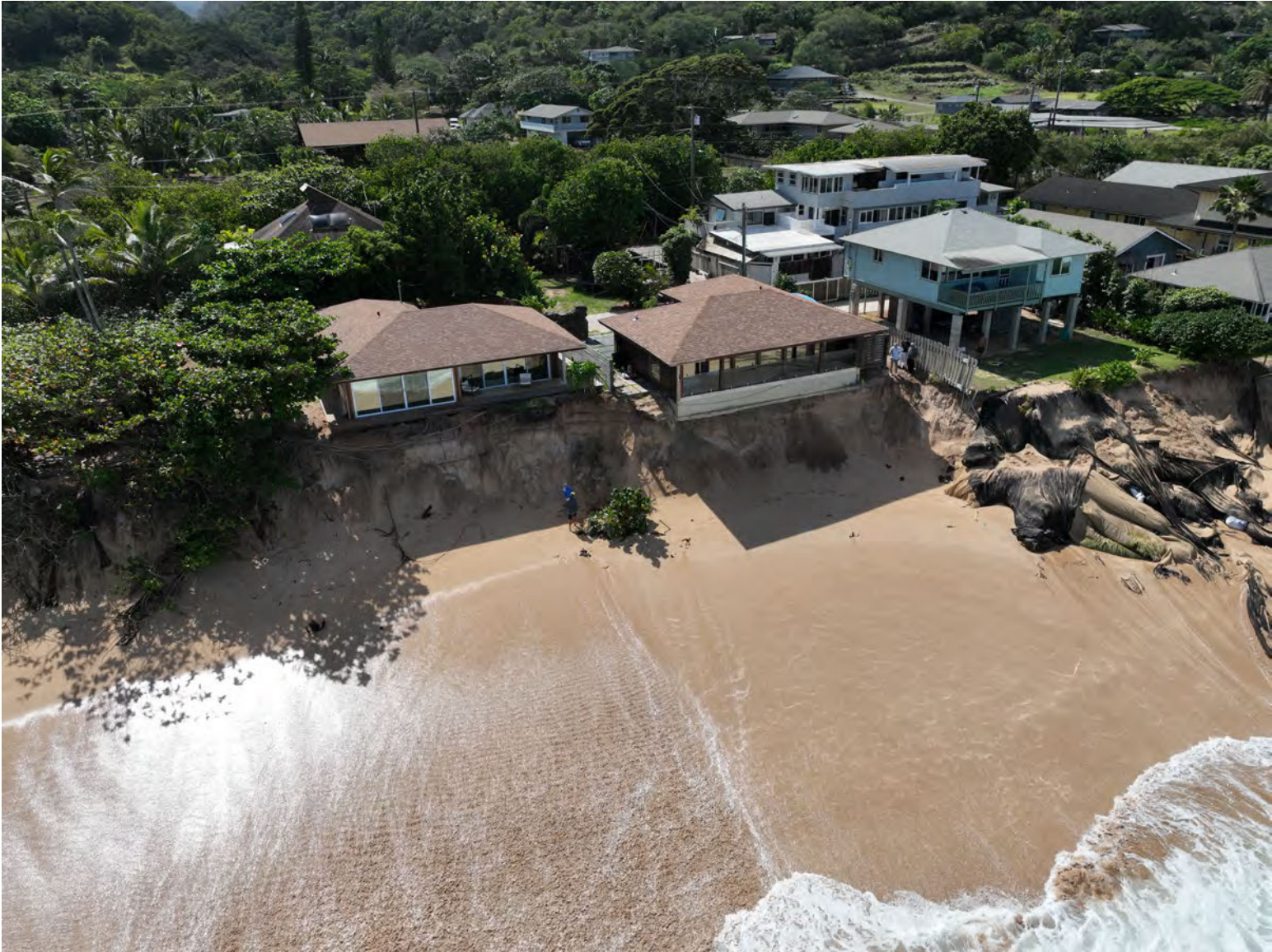
October 2, 2023 OCCL Photo of Shoreline Area Fronting Subject Parcel
