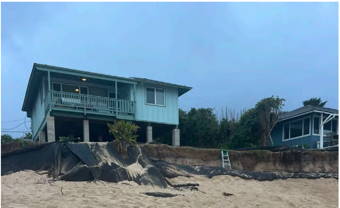
November 4, 2023 : Photo of shoreline area fronting subject parcel
