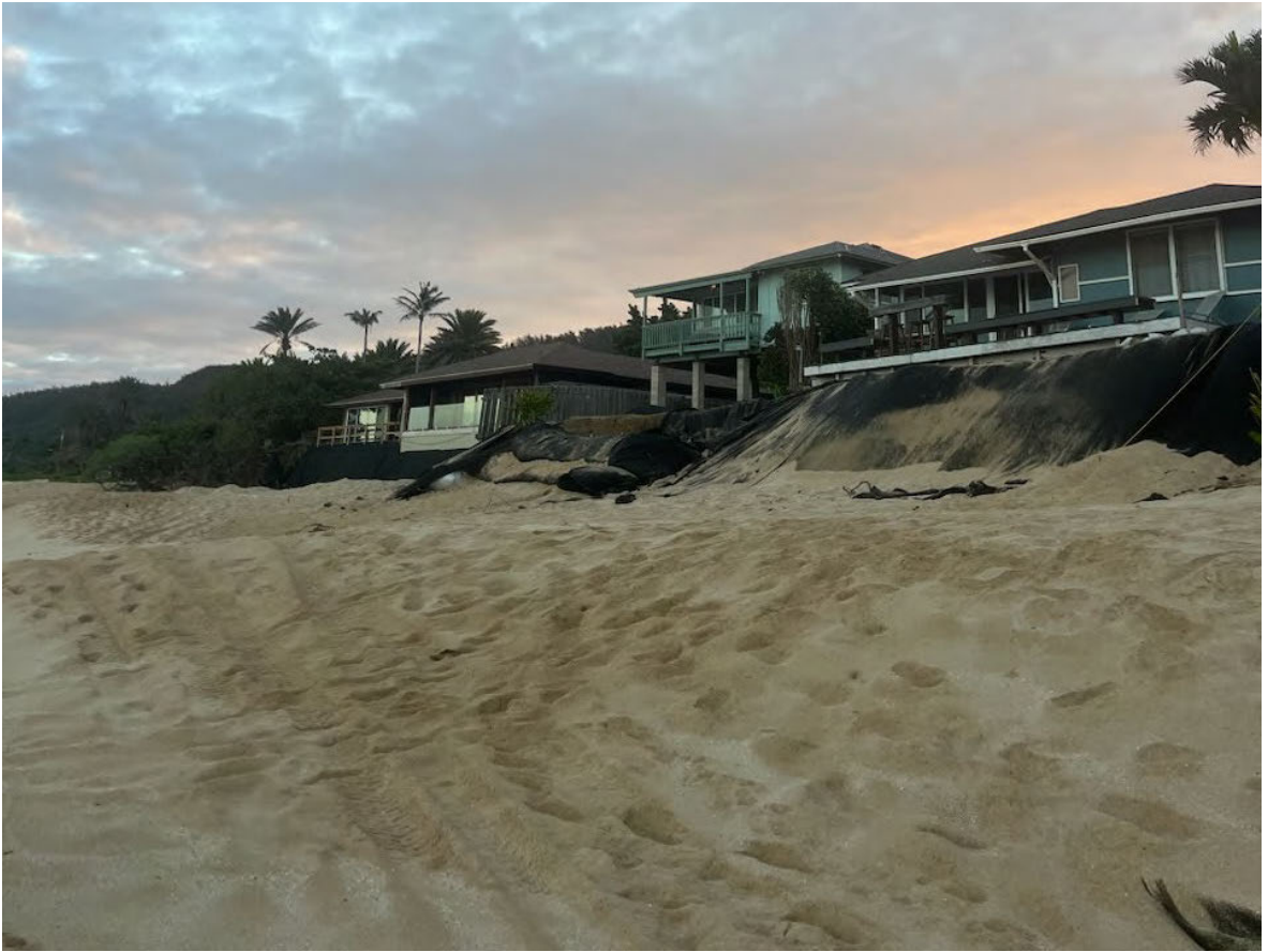
November 5, 2023 : Photo of shoreline area fronting subject parcel
