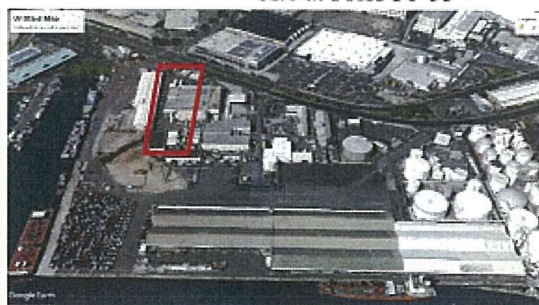
Site at Piers 31-33
