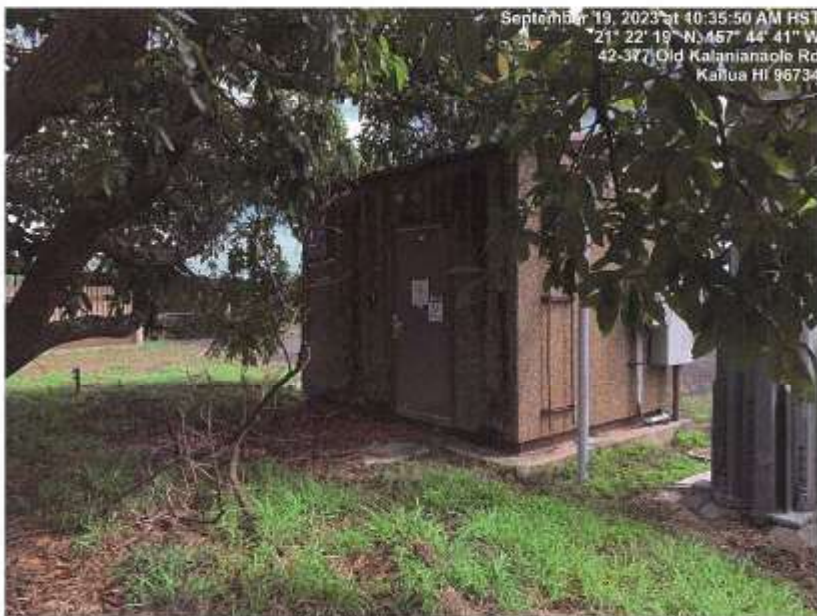
Figure 6: Doorway to structure within Easement A
