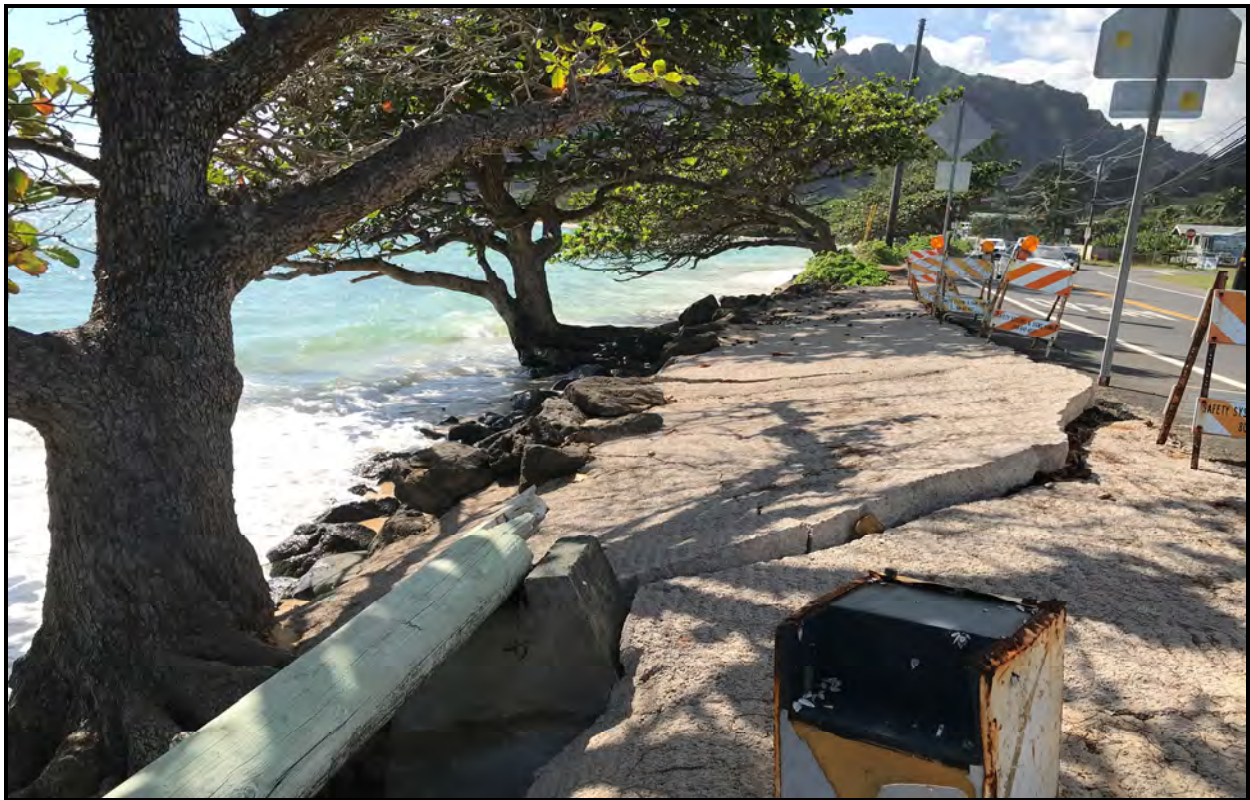
View of failed temporary revetment and narrowed Kaaawa beach.
