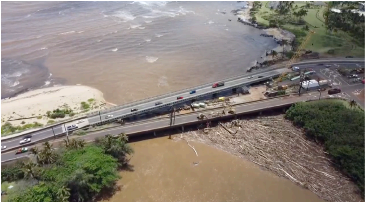
2024 - Wailua River half blocked by construction dam that caught timber debris.
