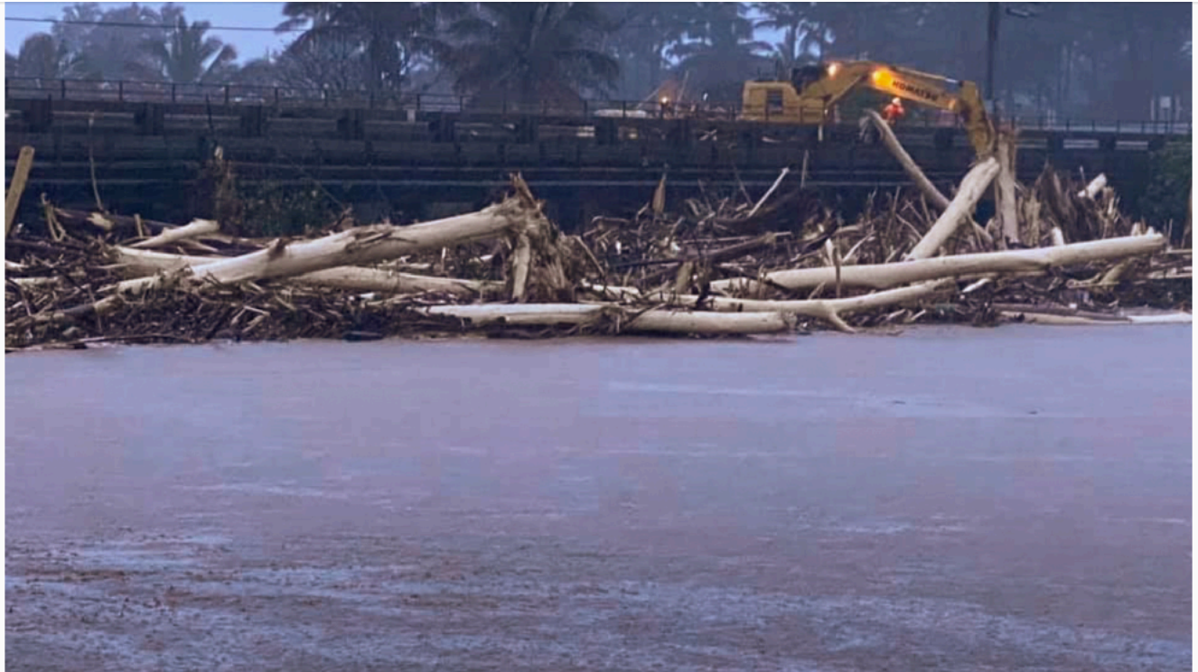
Fallen albizia limbs and branches washed down from the mountains during the rains of March 2020, which damaged the Wailua Bridge
