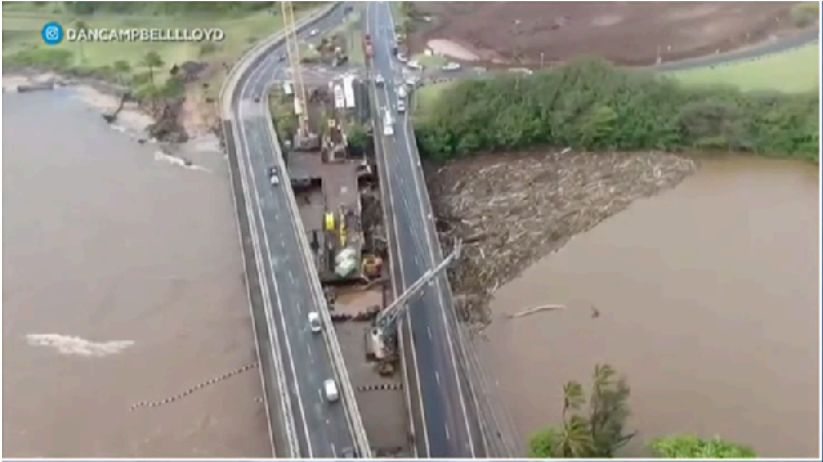
2024 - Wailua River half blocked by construction dam that caught timber debris.
