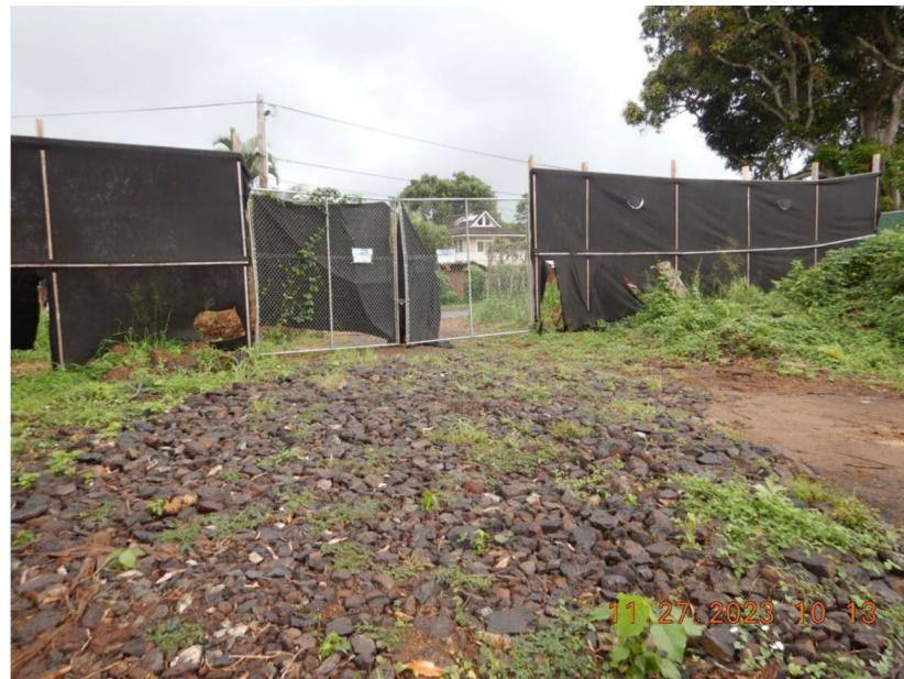
Photograph 12: View, facing northwest, of the third construction entrance located off Apana Road. Photograph taken by Rande Tubal on November 27, 2023.
