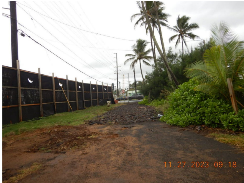
Photograph 11: View, facing south, of the second construction entrance located off Kuamoo Road. This entrance is approximately 20 m east of the entrance pictured in Photograph 1. Kuhio Highway is located on the other side of the dust screen. Photograph taken by Rande Tubal on November 27, 2023.
