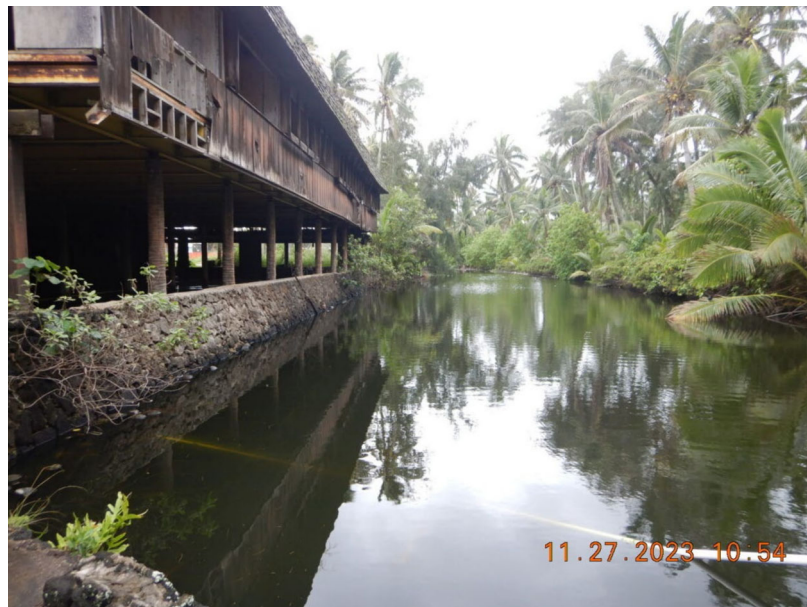
Photograph 4: View, facing south, of the Weuweu kawai iki fishpond. Note that the building pictured on the left is one of the buildings that will be undergoing construction. Photograph taken by Randee Tubal on November 27, 2023.
