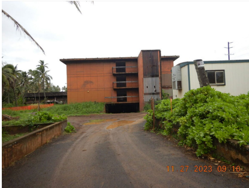
Photograph 13: Wide view, facing north, of Building 1. Note the construction trailer located to the right of the photograph. Photograph taken by Rande Tubal on November 27, 2023.
