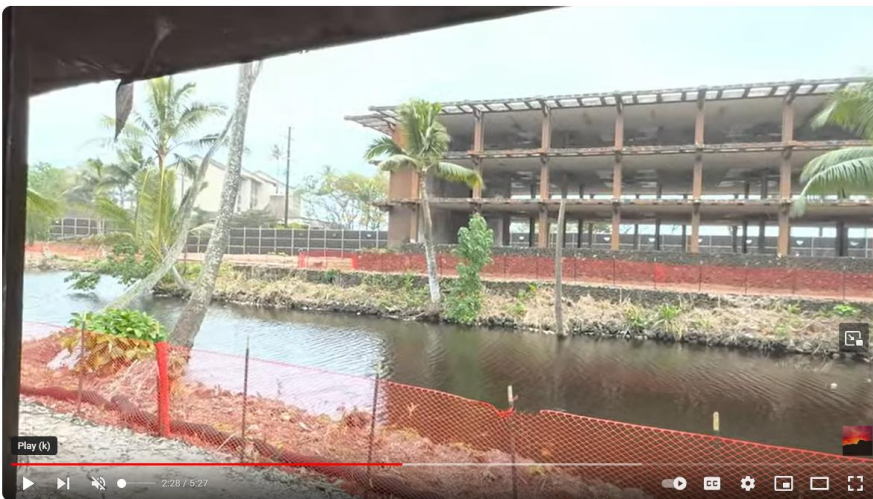
Coco Palms Demolition Part 2
