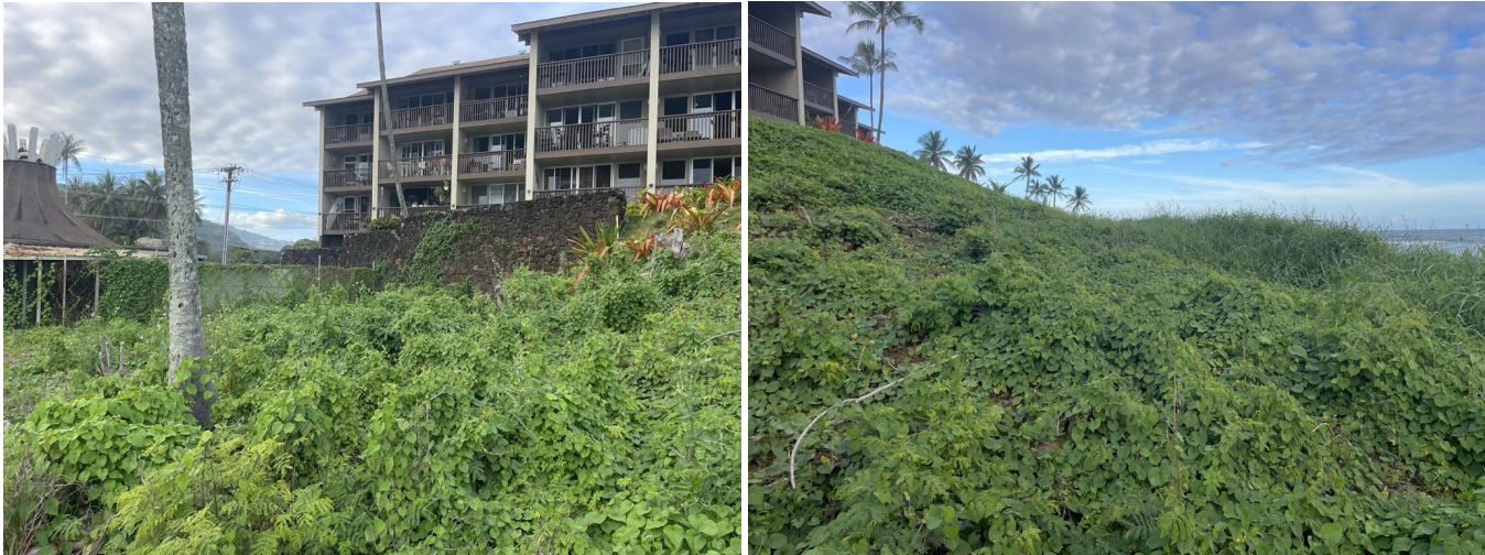
Images: View of the State parcel plateau area overlooking Wailua, covered with invasive vines/weeds.
