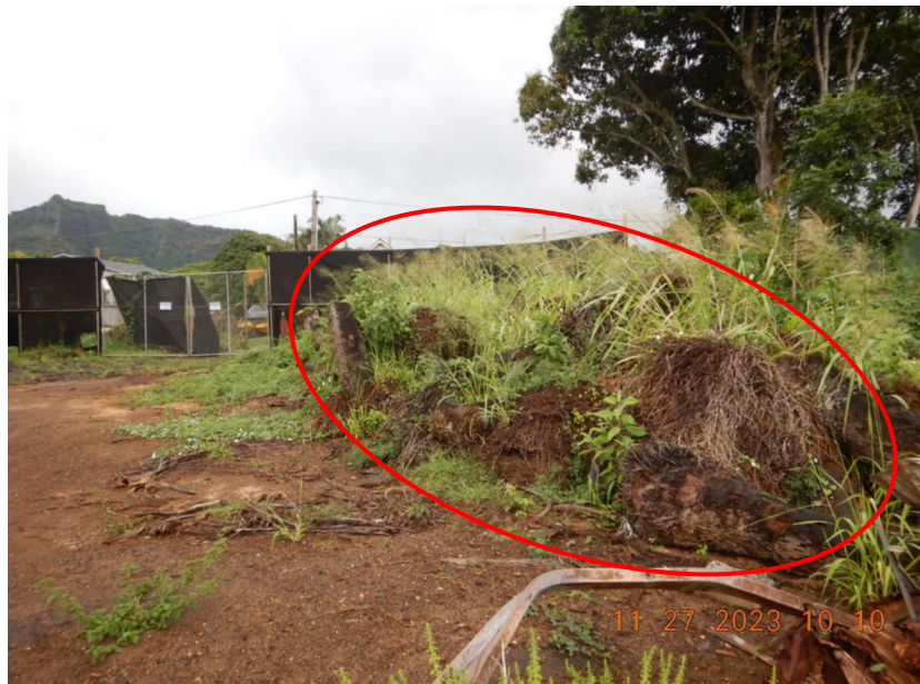
Photograph 20: View, facing north, of more coconut tree roots (stored on the northern end of Parcel 7). Note the Apana Street construction entrance in the background. Photograph taken by Rande Tubal on November 27, 2023.
