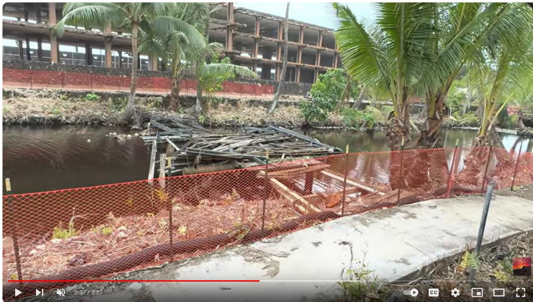
Coco Palms Demolition Part 2
