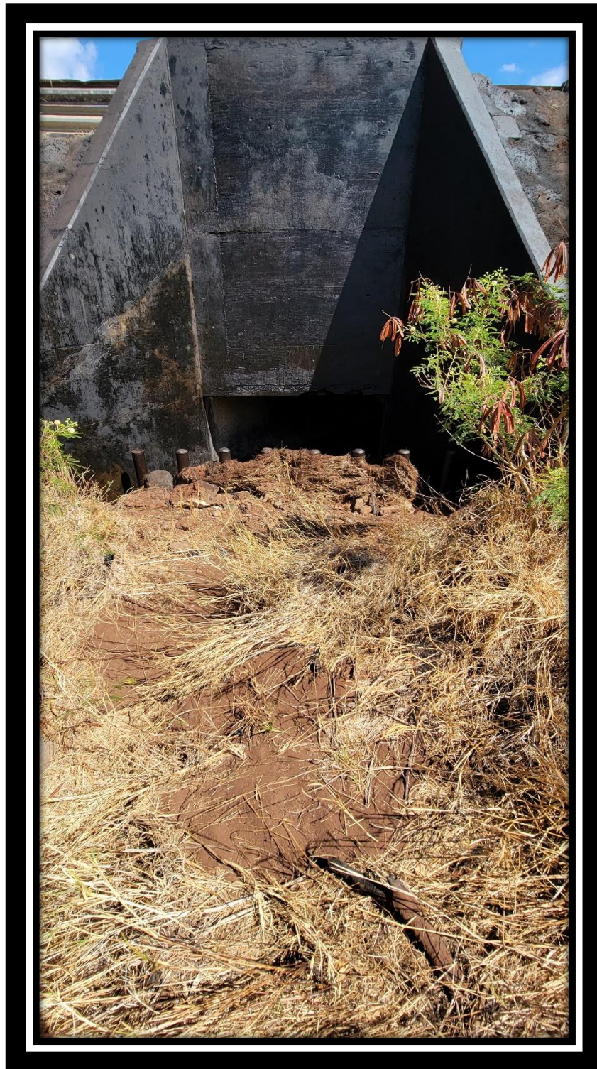
Figure 4 Gulch Facing Makai at the Storm Drain Ingress
