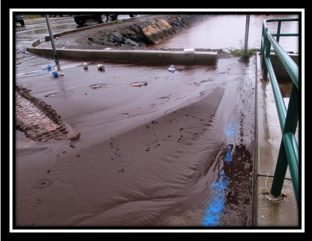
Figure 6 Sedimentation Overflow Ma'alaea Harbor at the Boat Ramp
