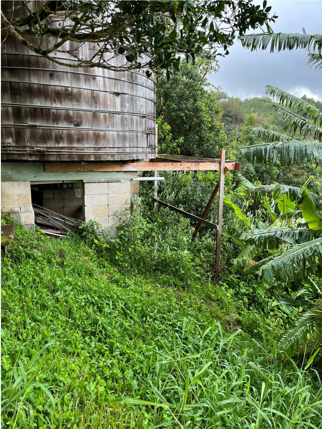
(Site #1, Existing Tank)
