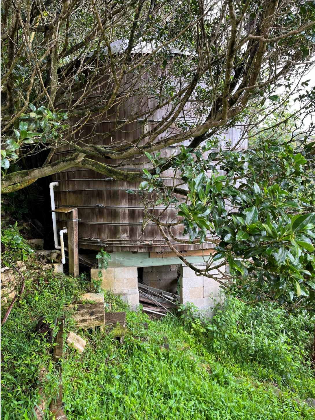
(Site #1, Existing Tank)
