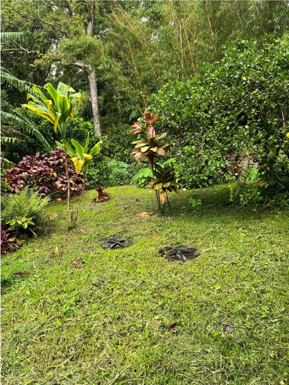
(Site #4, Septic Tank)
