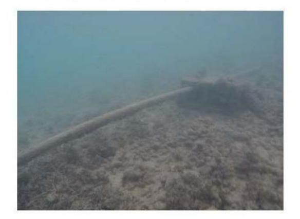
The photo below shows Resorttrust's abandoned PVC water pipe sticking up from the ocean floor approximately 6' feet deep, between the Western groin and the islet. At low tide this pipe extends out of the water as shown in the photo and is a hinderance to swimmers in the lagoon.
