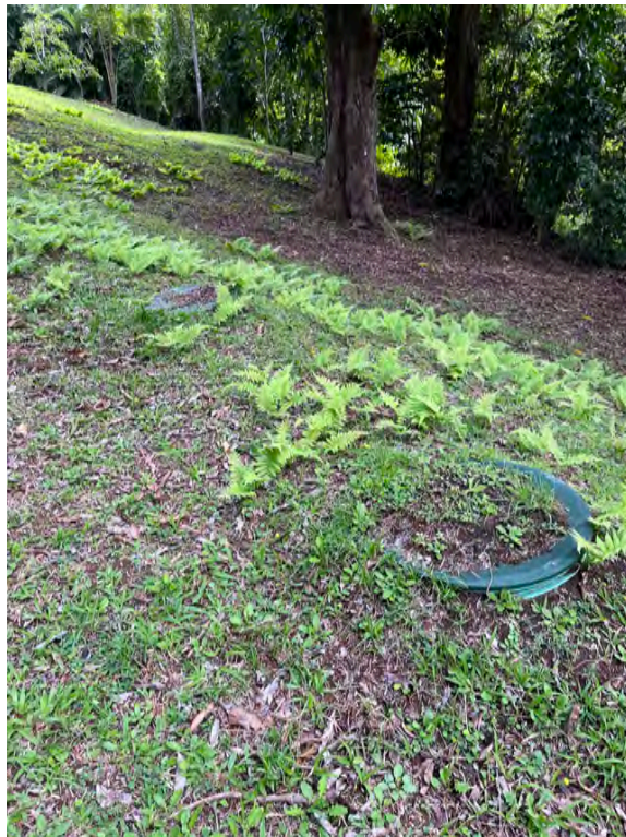
03/20/2024 OCCL photo of septic system on Parcel 026
