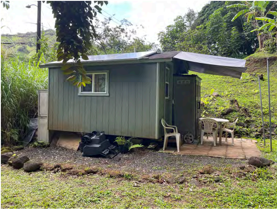
03/20/2024 OCCL photo of shed, solar panel(s), storage cabinets, covered lanai/porch
