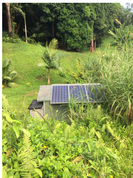
11/02/2018 OCCL photo of Parcel 026 and shed with solar panels and storage cabinet
