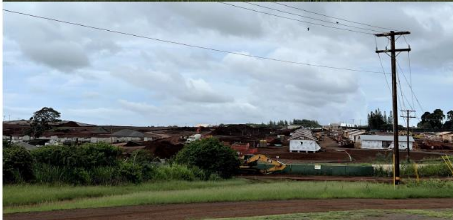
Hōkūau Residential Development under construction
