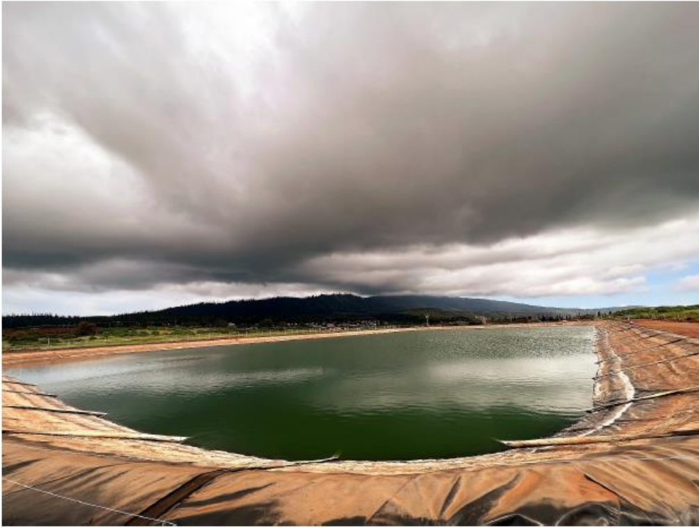
Lānaʻi City Auxiliary Reclamation Facility Pond
