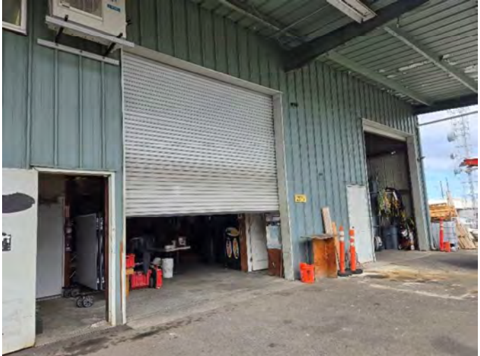
Last two bays at rear of building.
