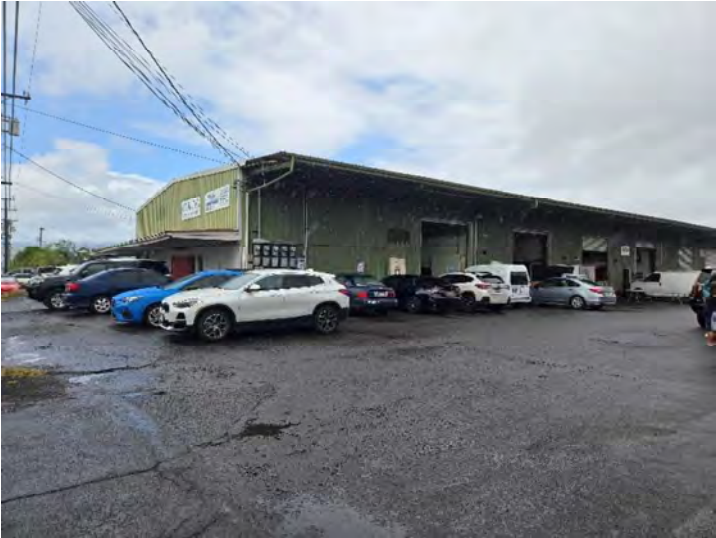
Building on left side of property. Note separate electric meters for each tenant.
