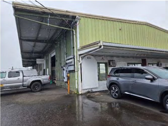
Building on right side of property. Note separate electric meters for each tenant.
