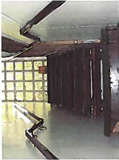
Depicts exterior exit stairway.
