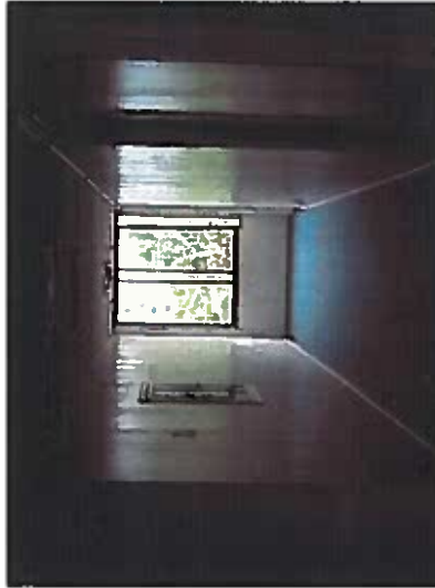
Depicts dead end corridor on the Makai wing on floors 2 thru 6.
