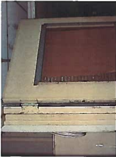
Depicts louvered door on second floor to telephone room.
