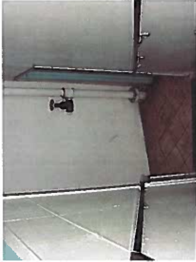
Depicts bottom of exit stairway. (directional illuminated exit sign required)
