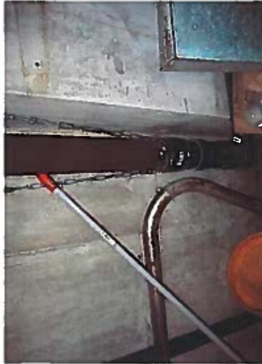
Photo of laundry waste pipe connection to sanitary drain pipe.
