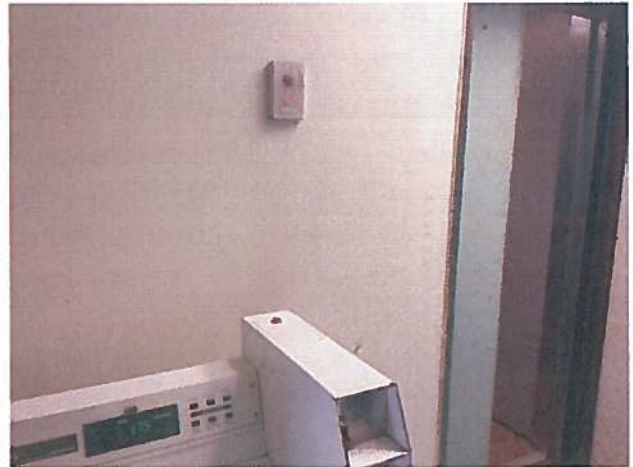
Pull station on elevator wall near rear of building blocked and painted *MANY PULL STATIONS WERE PAINTED*
