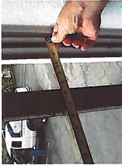
Depicts widow openings greater than 4 inches and the grade below is over 72 inches from the bottom of the opening.
