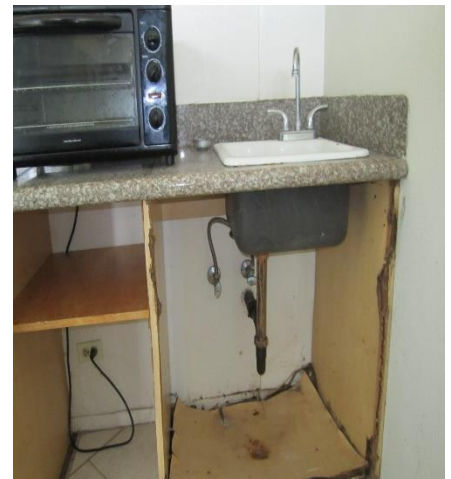
Photo of Kitchen Sink installed opposite side of wash basin.
