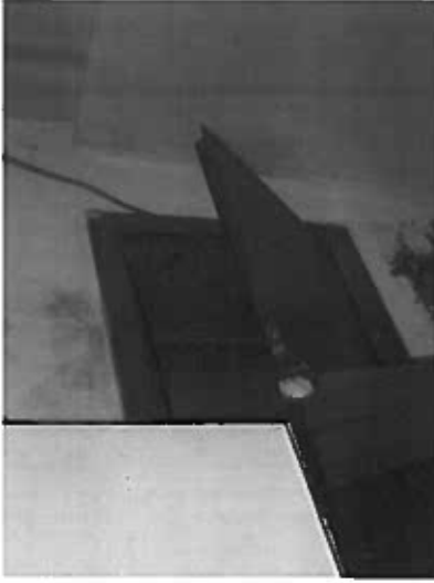
Depicts laundry shoot door open. (door is required to be self-closing)
