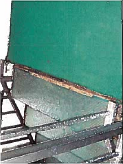
Depicts spacing between the exit stairs and landing.
