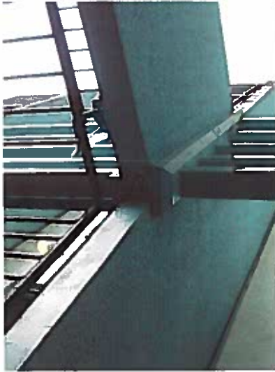
Depicts deteriorating concrete walkway supported by wood structural members. (wood material used in type IB construction must be heavy timber and have a fire-resistance rating of 2 hours)
