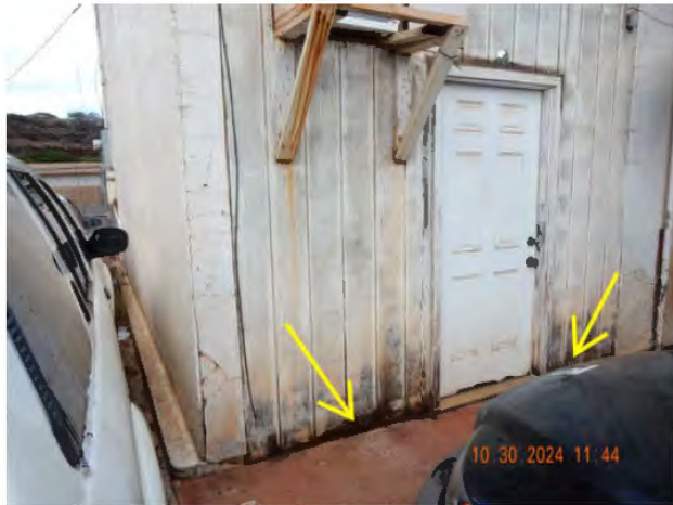
Figure 34. Exterior wood wall (DSCN3887).
