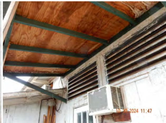
Figure 46. Exterior painting (DSCN3917).
