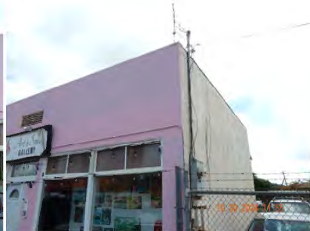
Figure 50. Exterior painting (DSCN3973).
