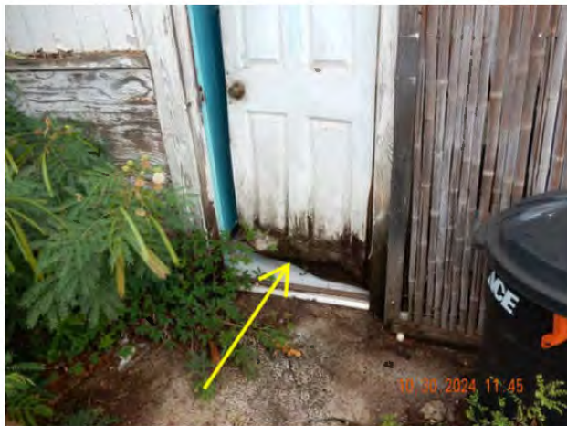
Figure 36. Exterior wood wall (DSCN3899).
