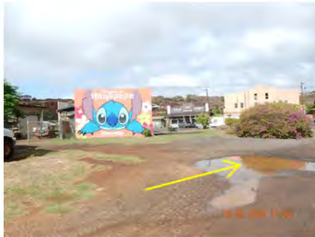
Figure 23. Low lying areas of property (DSCN3711).
