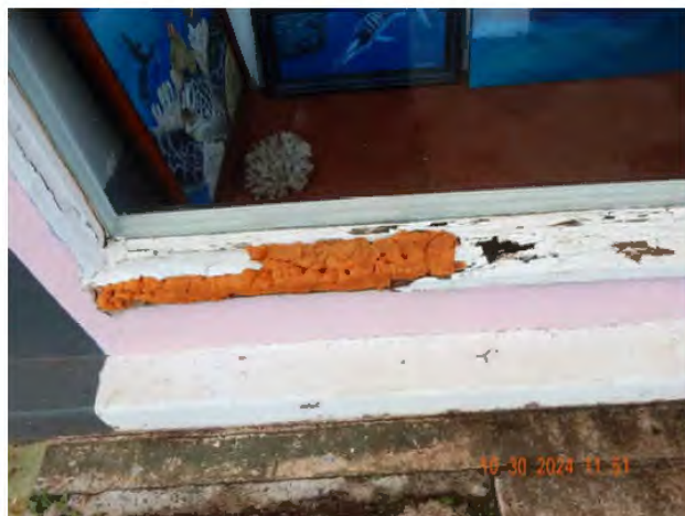
Figure 38. Exterior wood wall (DSCN3944).
