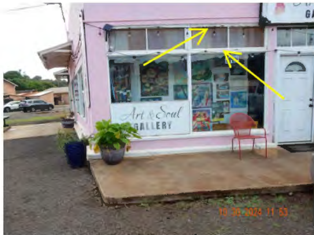
Figure 40. Exterior wood wall (DSCN3960).
