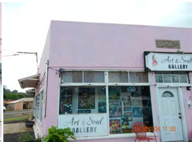
Figure 48. Exterior painting (DSCN3959).
