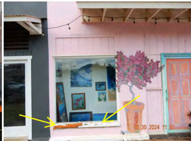
Figure 37. Exterior wood wall (DSCN3942).
