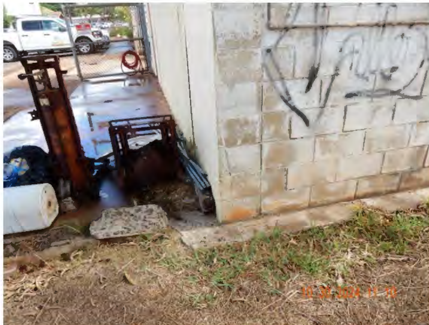
Figure 71. Unwanted materials around building (DSCN3726).
