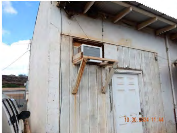
Figure 43. Exterior painting (DSCN3888).
