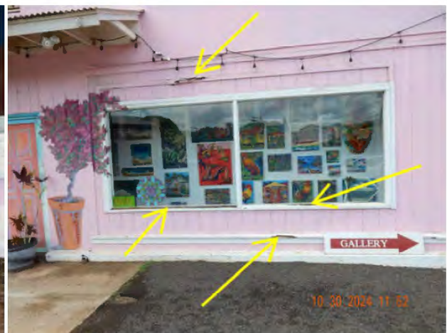
Figure 39. Exterior wood wall (DSCN3952).
