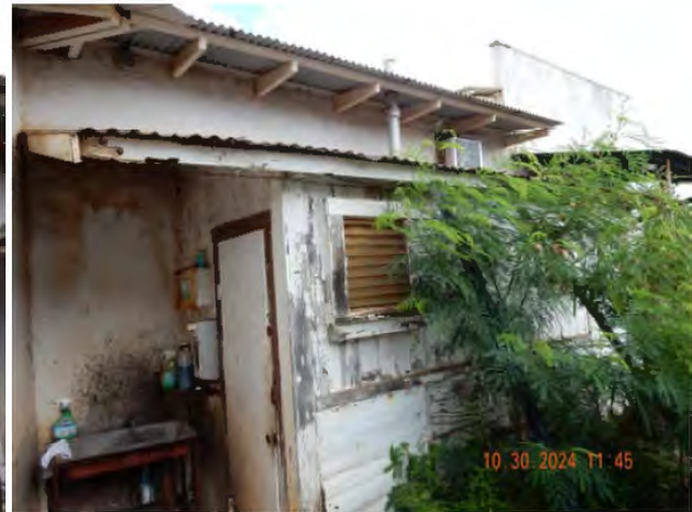
Figure 44. Exterior painting (DSCN3895).
