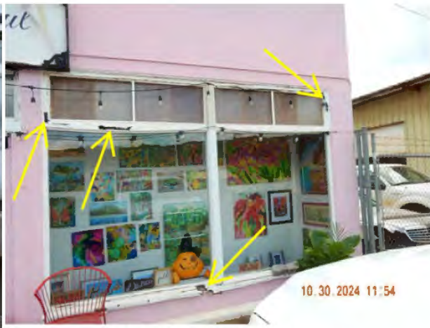
Figure 41. Exterior wood wall (DSCN3967).
