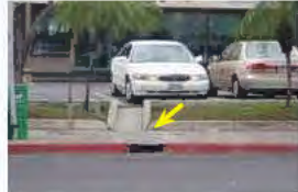
Sidewalk culverts are storm drain connections.
