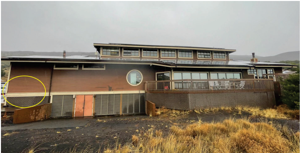
Fig. 2. South-facing wall of HP common building. Circled area shows where solar collectors will be secured between concrete pad and outer wall. Red double doors indicate entry to Mechanical Room.
