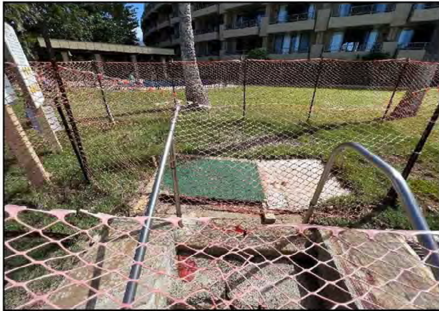
Figure 13. Covered sinkhole at top of north stairway
