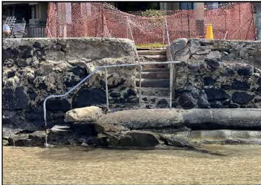
Figure 12. Concrete/mortar bags located on the north end with undermining at the toe
