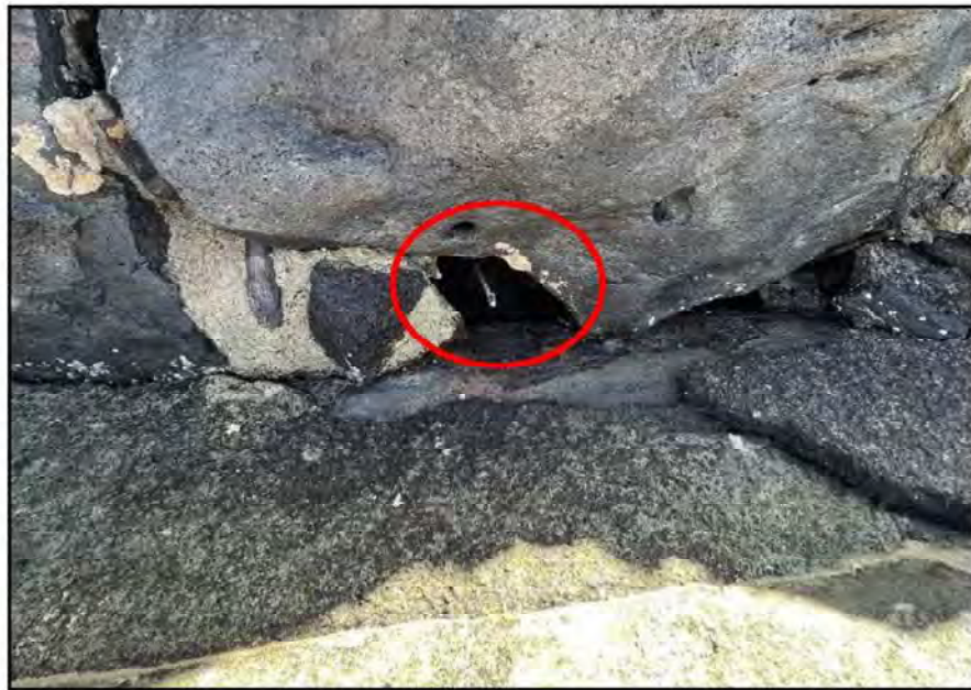
Figure 9. Survey rod inserted into CRM wall to a depth of 3 feet (circled in red)
