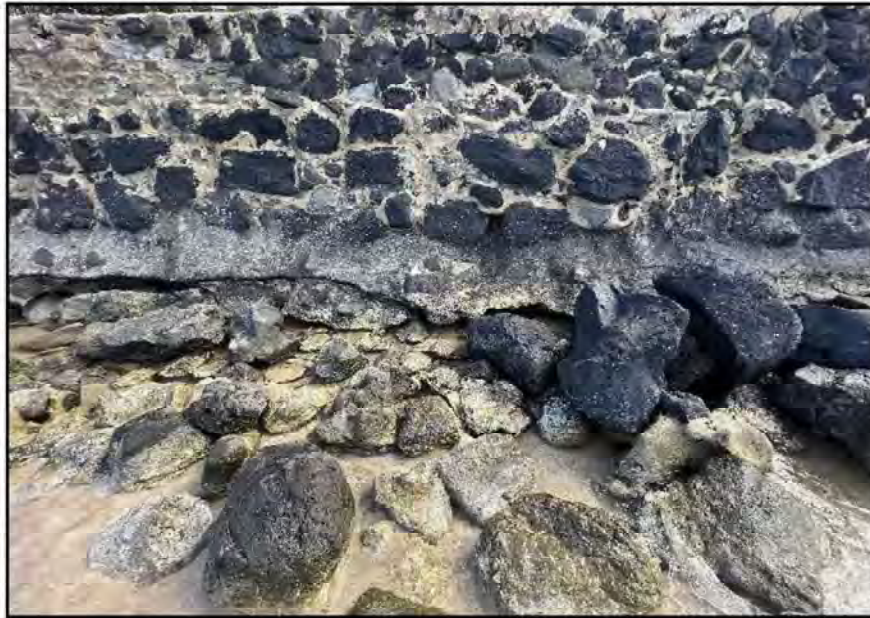
Figure 11. Stones at the base of the wall with various stages of mortar and grout conditions
