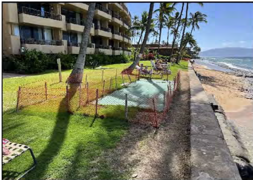
Figure 14. Covered sinkhole south of north stairway
