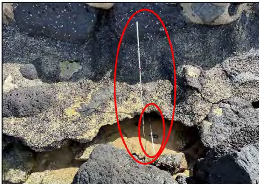
Figure 8. North section of wall undermining, 3-foot survey rods (circled in red)
