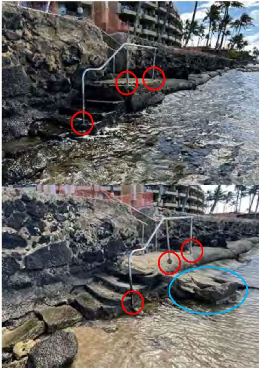
Figure 5. North stairway (November 8, 2021, railing (top circled in red) connected to landing and February 8, 2023, railings (bottom circled in red) not connected to landing which has fallen onto the shoreline (bottom circled in blue), looking southeast)
