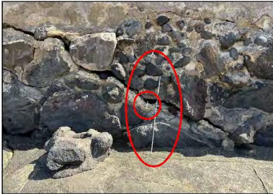
Figure 7. Diagonal crack in wall above concrete/mortar bags, 3-foot survey rods (circled in red) one inserted into crack to an approximate depth of 2 feet
