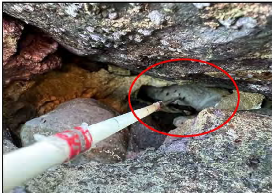
Figure 10. Soft foam structure behind CRM wall at tip of survey rod (circled in red)
