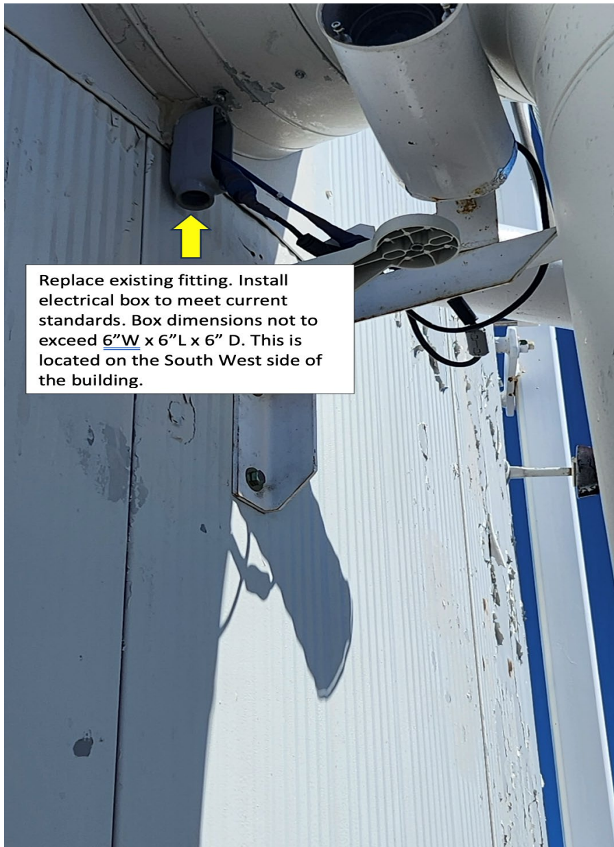
Figure 4. Southwest corner needing conduit box.
