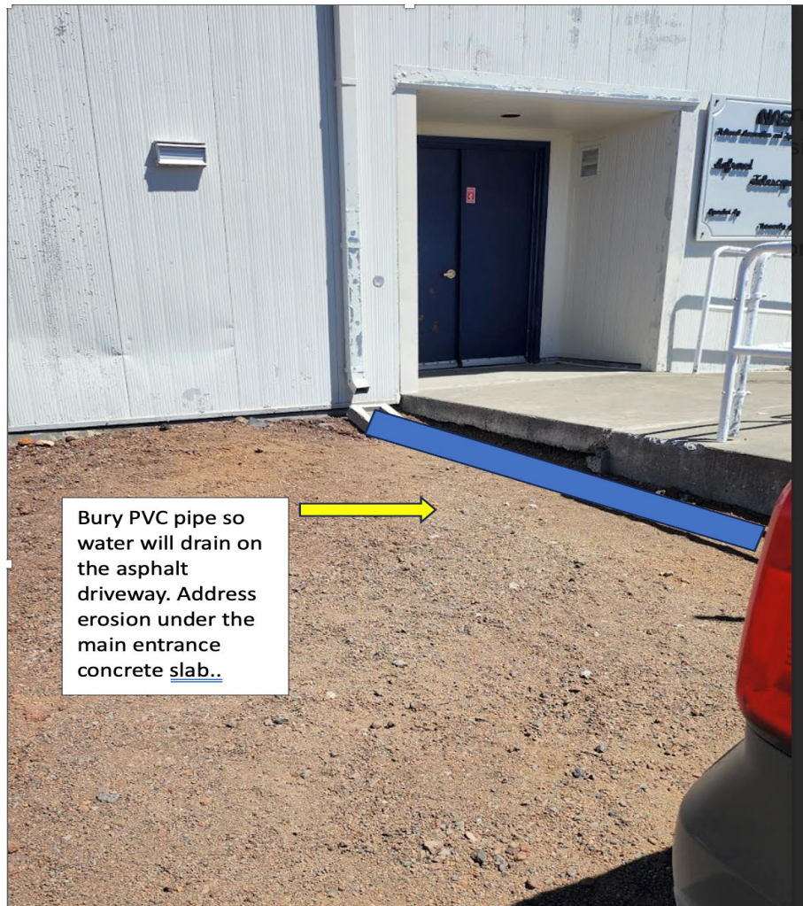
Figure 1. PVC pipe will not be 'buried,' but covered over by fresh cinder between the building to the beginning of the asphalt (flush with rear end of vehicle to right of image).
