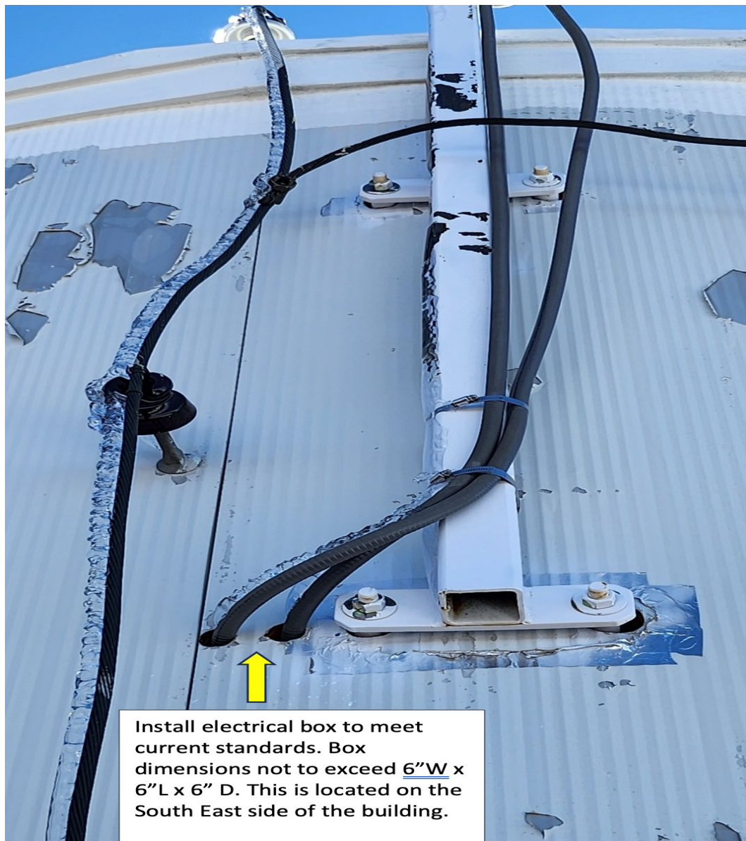
Figure 5. Southeast corner needing conduit box.
