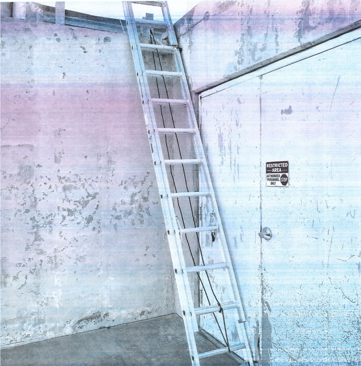
Figure 1 - The existing ladder (photographed by the Maunakea Rangers). The replacement ladder would mount to the wall, but otherwise in a similar location.
