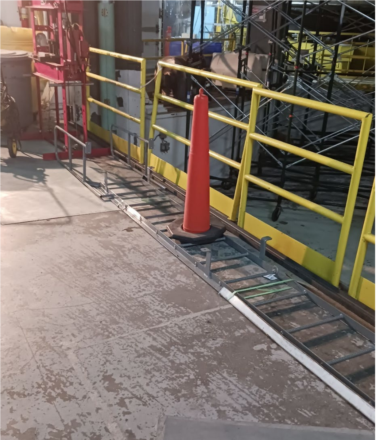
Figure 2 - Replacement ladder: the steel structure lying horizontally. The top-end safety hand rails are to the upper left in this image. These will be above the upper wall edge on the left in Figure 1.
