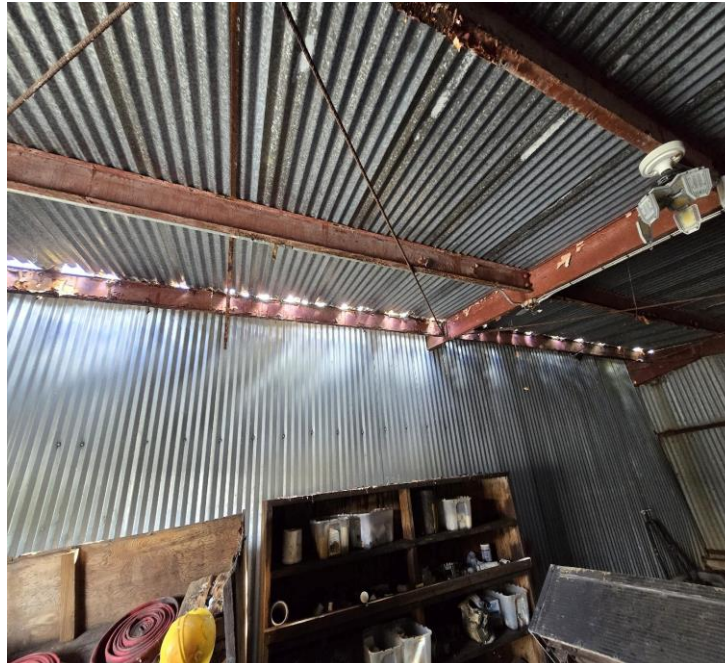
Chemical room requires new roofing.
