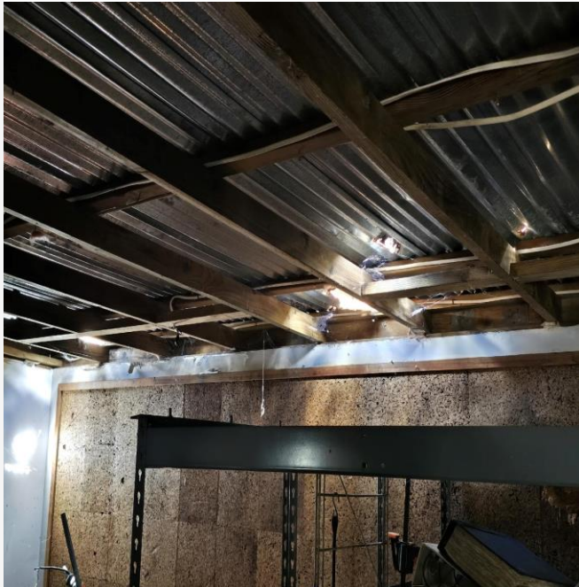
Mechanical room requires new roofing
