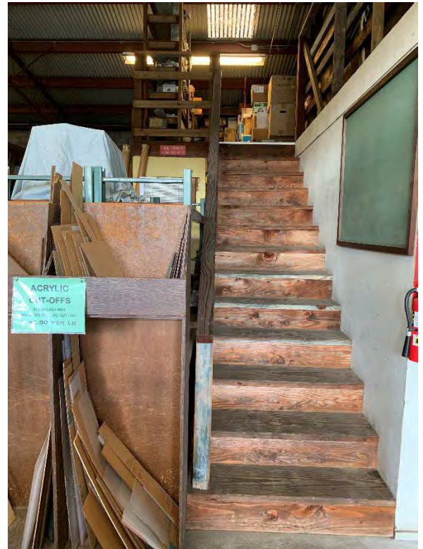
MEZZANINE ACCESS STAIRS
