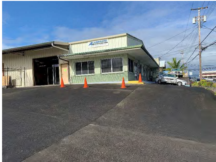
FRONT OF BUILDING FROM STEEP DRIVEWAY. RETAIL, CUSTOMER SERVICE AND OFFICE AREAS IN GREEN PORTION. WAREHOUSE AREA BEGINS AT BAY DOOR.
