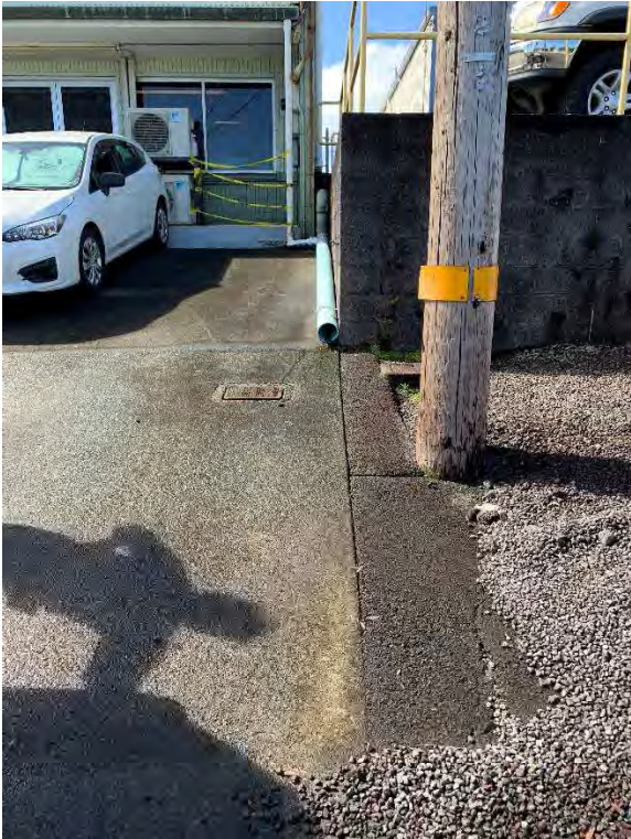
SHARED ROOF DRAINAGE TO STREET
