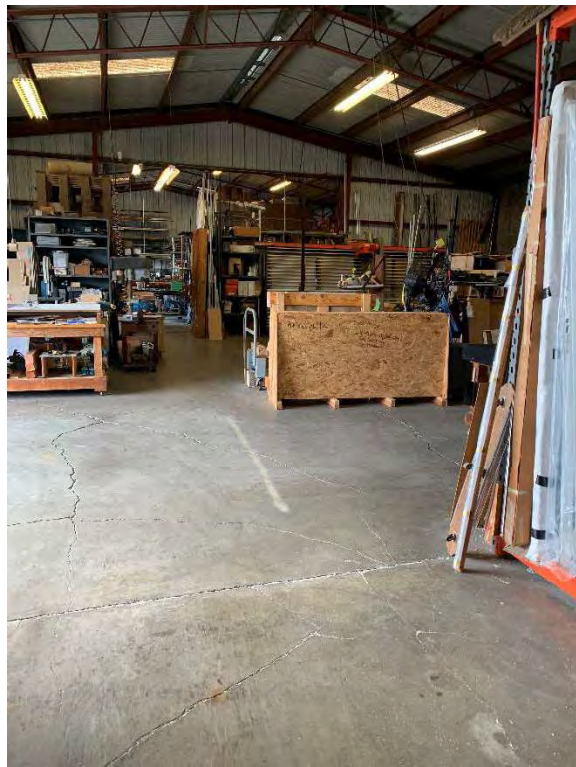
VIEW OF BACK OF ORIGINAL WAREHOUSE. NOTE STRESS CRACKS IN FLOOR. WALL IN BACKGROUND IS END OF ORIGINAL WAREHOUSE
