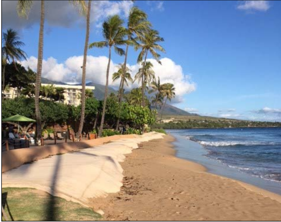
Figure 3-4 Erosion protection skirt (Kaanapali, Maui, Hawaii)
