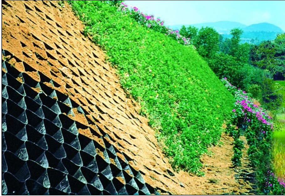
Figure 3-3 Slope stabilization with vegetation and GEOWEB
