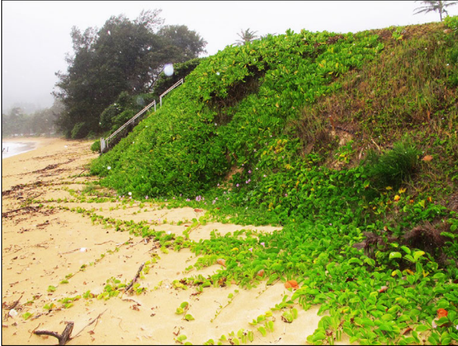
Figure 2-10 Previous condition of the shoreline, looking south (6/13/2013)
