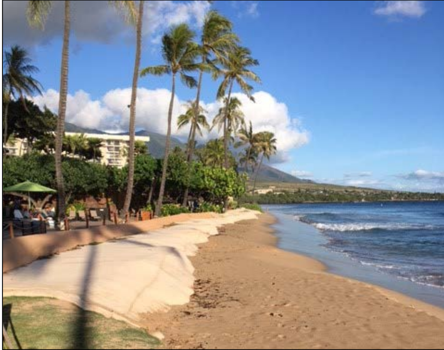
Figure 3-4 Erosion protection skirt (Kaanapali, Maui, Hawaii)
