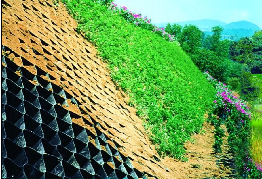
Figure 3-3 Slope stabilization with vegetation and GEOWEB
