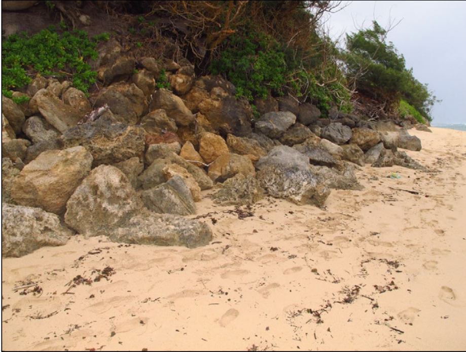
Figure 2-4 Northern portion of the Muliwai shoreline (6/13/2013)
