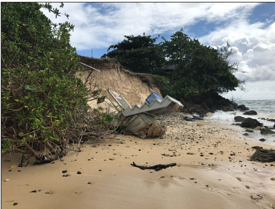
Figure 2-9 Current condition of the shoreline, looking north (7/19/2017)
