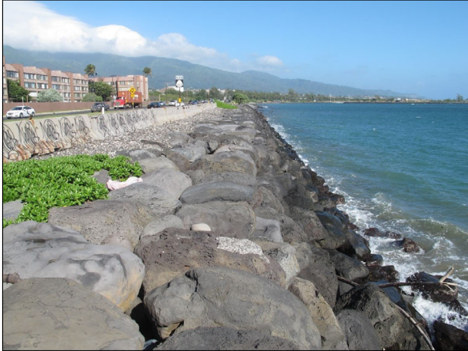
Figure 3-9 Typical rock revetment (Kahului, Maui, Hawaii)
