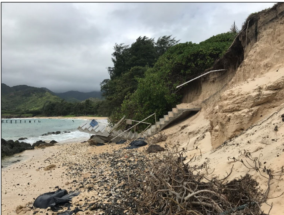
Figure 2-11 Current condition of the shoreline, looking south (7/19/2017)
