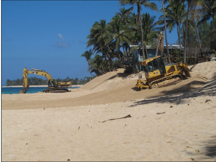
Figure 3-1 Sand pushing (Sunset Beach, Oahu, Hawaii)
