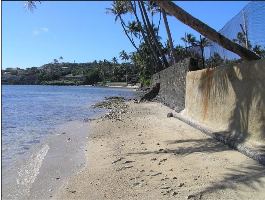
Figure 3-8 Typical concrete and rock seawalls (Kahala, Oahu, Hawaii)
