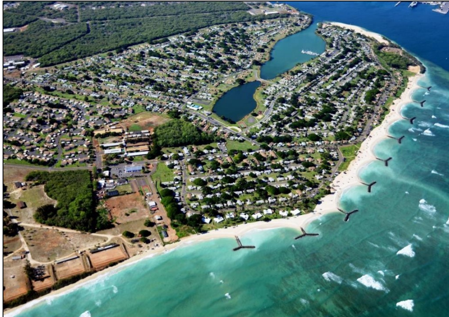
Figure 3-7 Beach nourishment with T-head groins (Iroquois Point, Oahu, Hawaii)
