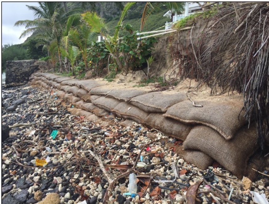
Figure 3-5 Biodegradable sandbag revetment (Waimanalo, Oahu, Hawaii)
