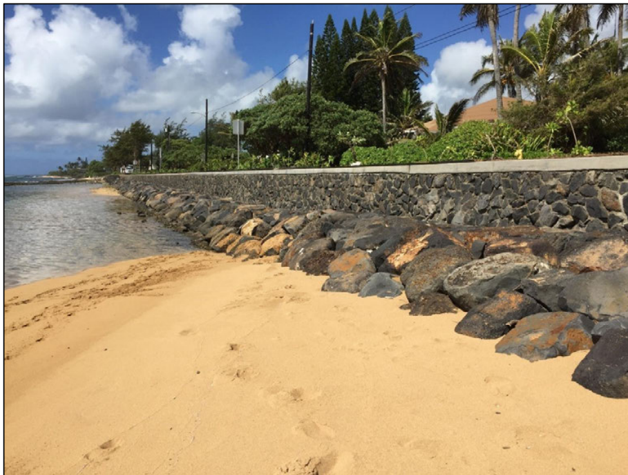
Figure 3-10 Hybrid Seawall-Revetment (Kapaa, Kauai, Hawaii)
