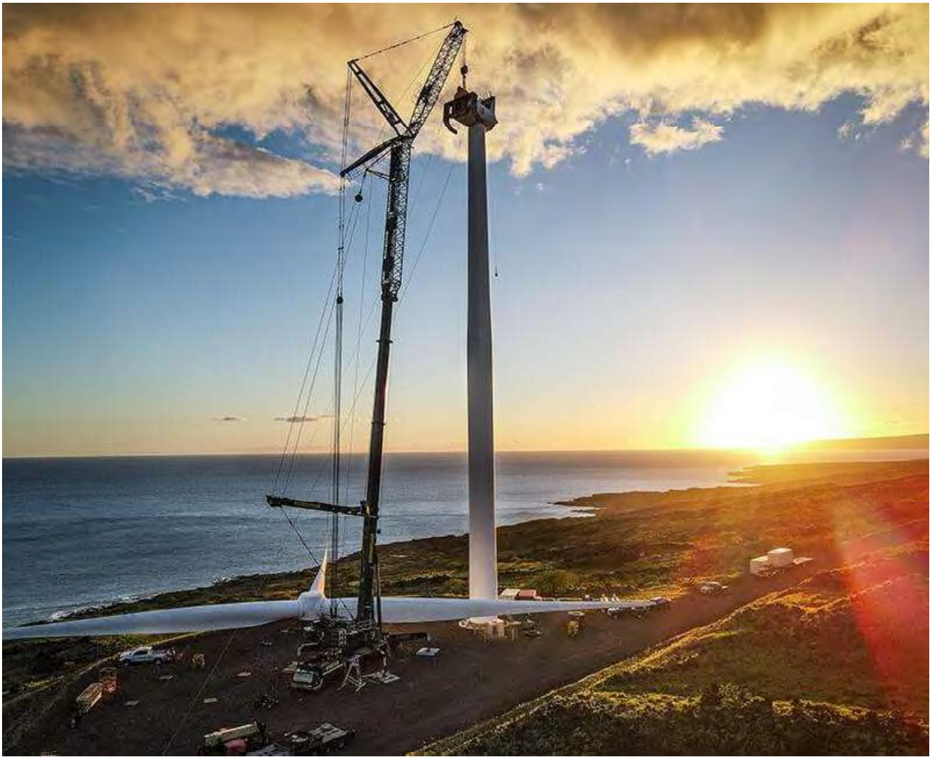
Figure C-2. Kaheawa Wind Power, Liebherr LTM 1150 Crane Operations (Source: Mountain Crane)
