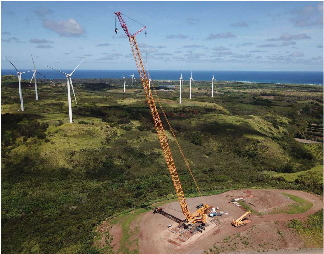
Figure C-1. Hawi Wind Farm, Liebherr LR11000 Crawler Crane Operations (Source: Buckner Heavy Lift)
