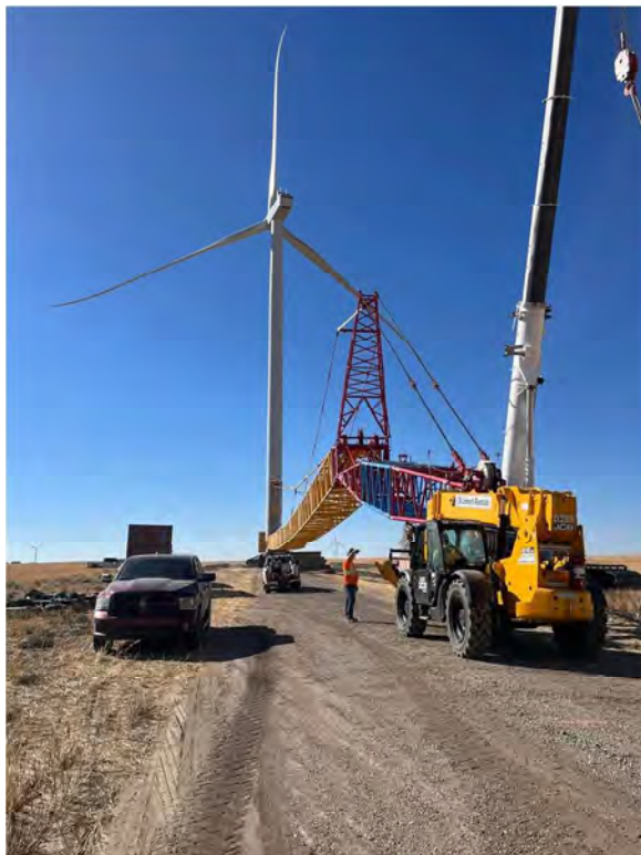
Figure C-19. Assembly of Liebherr LR 11000 Crawler Crane (Source: Buckner Heavylift)
