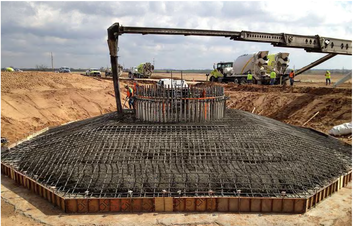
Figure C-22. Typical Wind Turbine Spread Footing (Source: https://www.windsystemsmag.com )
