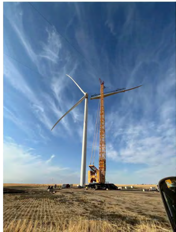
Figure C-20. Assembly of Liebherr LR 11000 Crawler Crane (Source: Buckner Heavylift)
