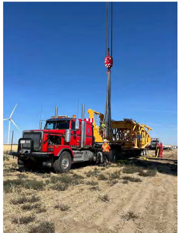
Figure C-13. Assembly of Liebherr LR 11000 Crawler Crane (Source: Buckner Heavylift)
