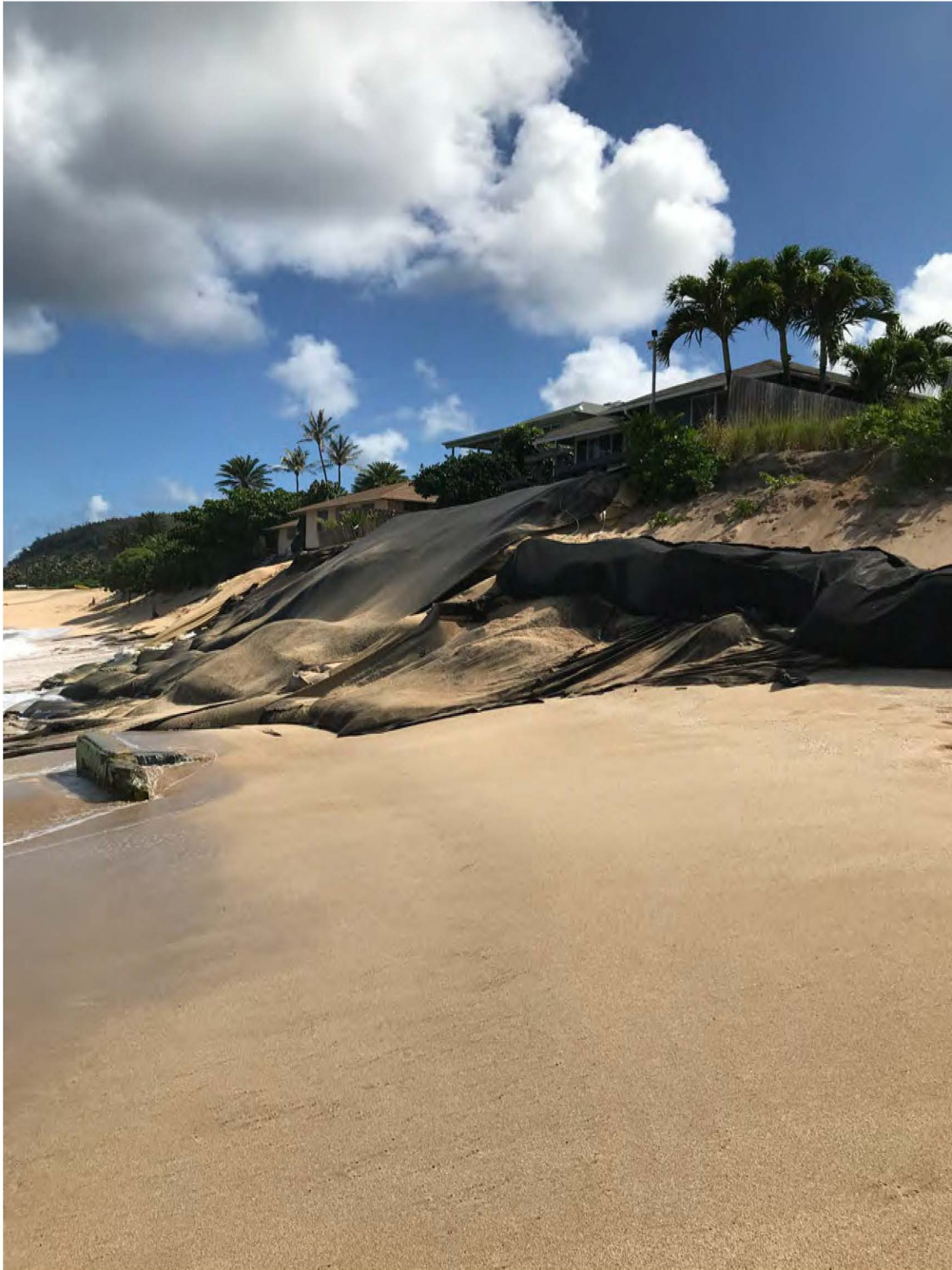
10/18/2021 Additional Unauthorized Work in the Form of an Erosion Control Blanket
