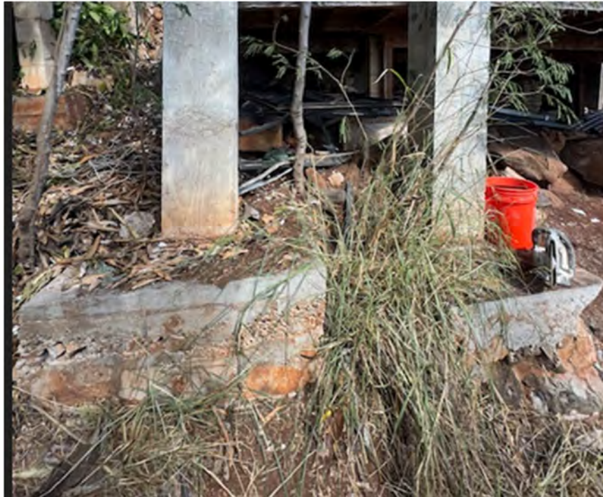
Storage of Large/Heavy Materials that Could Not be Removed During Additional Removal and Cleanup
