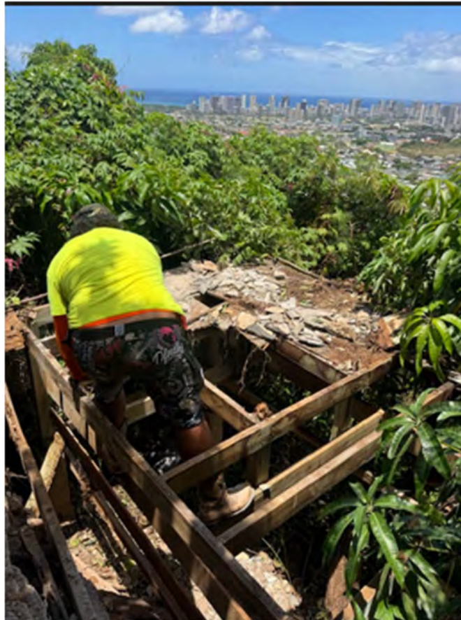
Alleged Encroachment (Deck) Removal - In Progress
