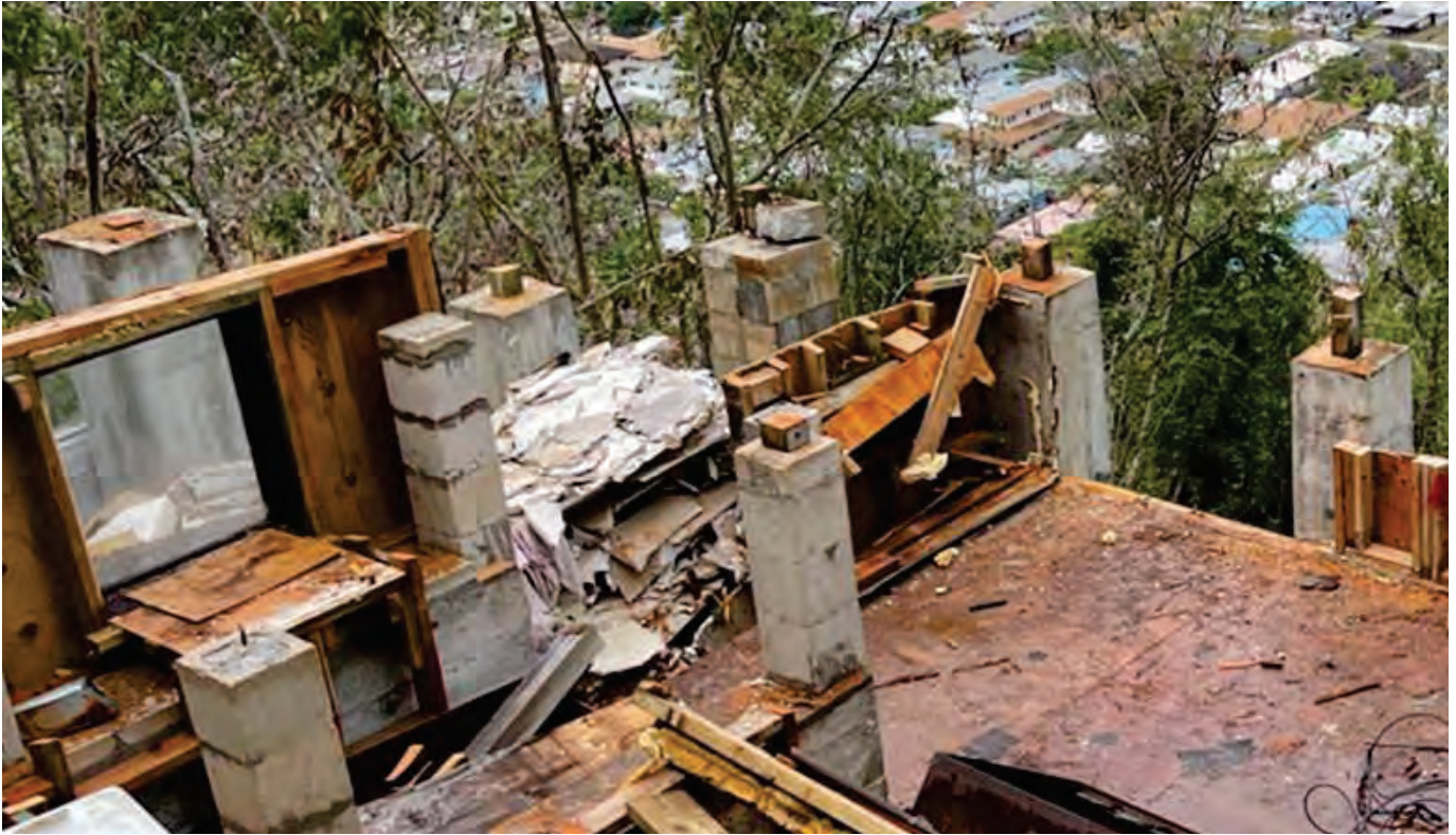
Second Floor Removed
