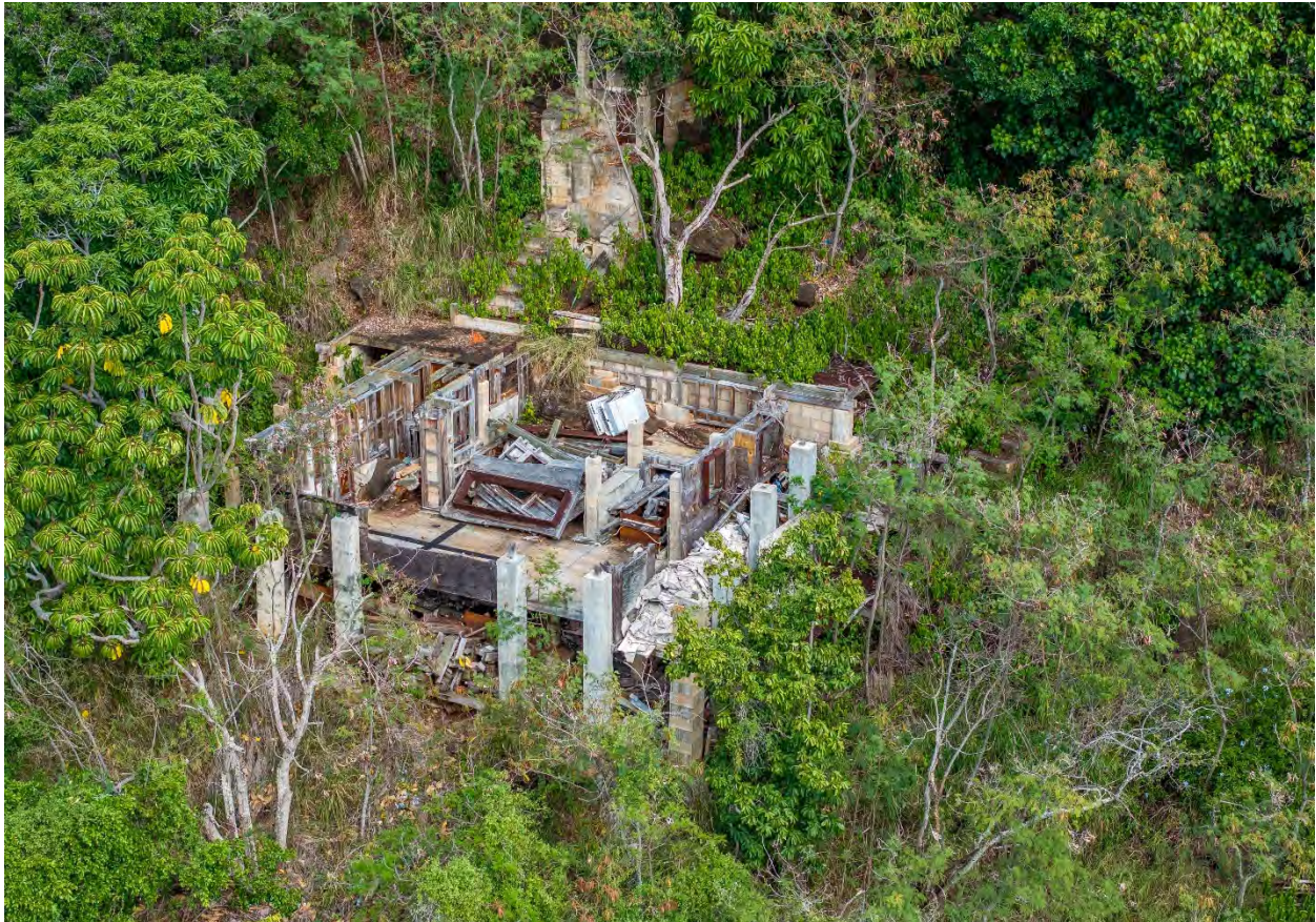
Shed Prior to Additional Removal and Cleanup
