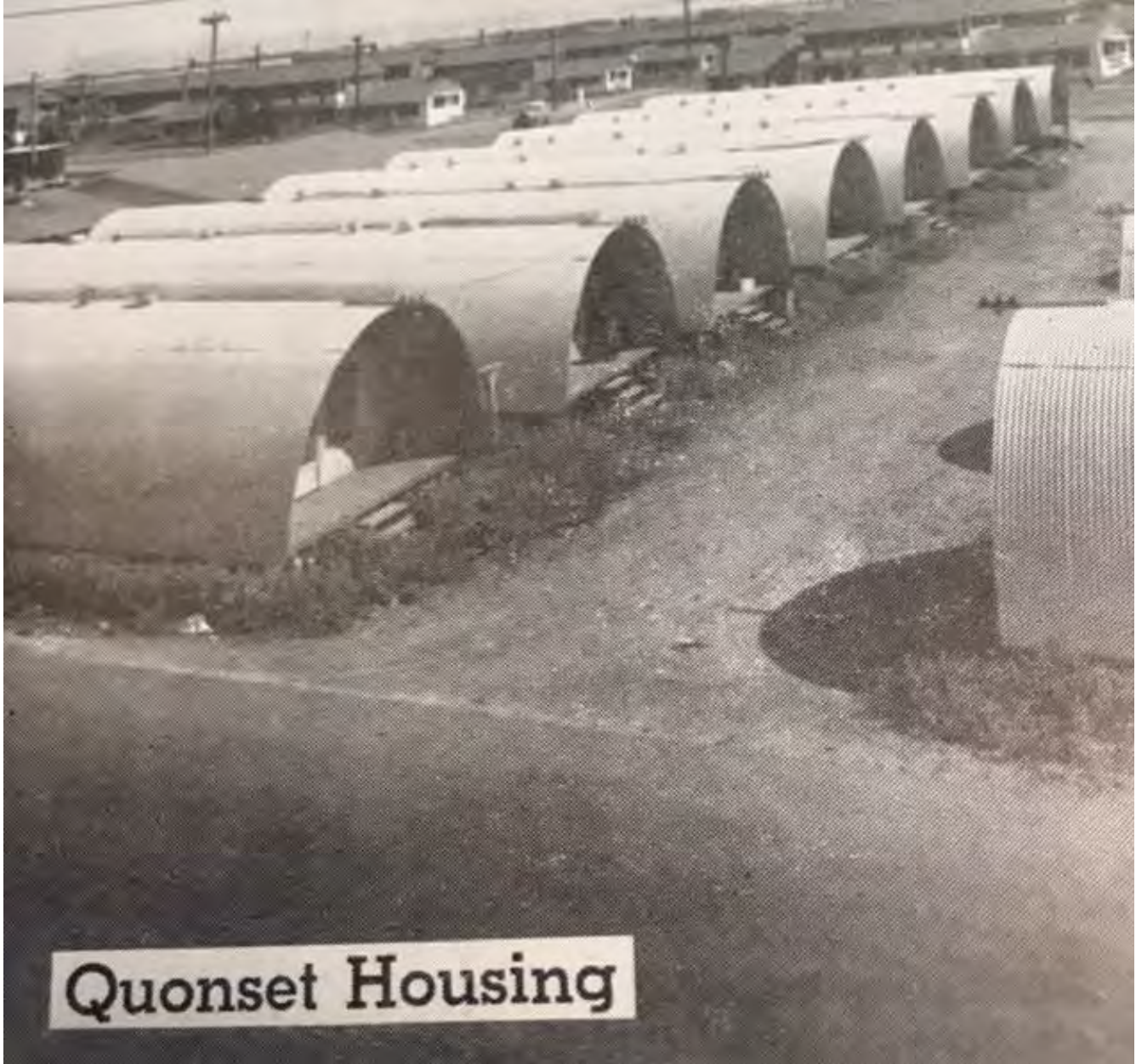
Figure 28. View of Quonset huts used as housing. Source: Navy Banner newspaper, 1943.
