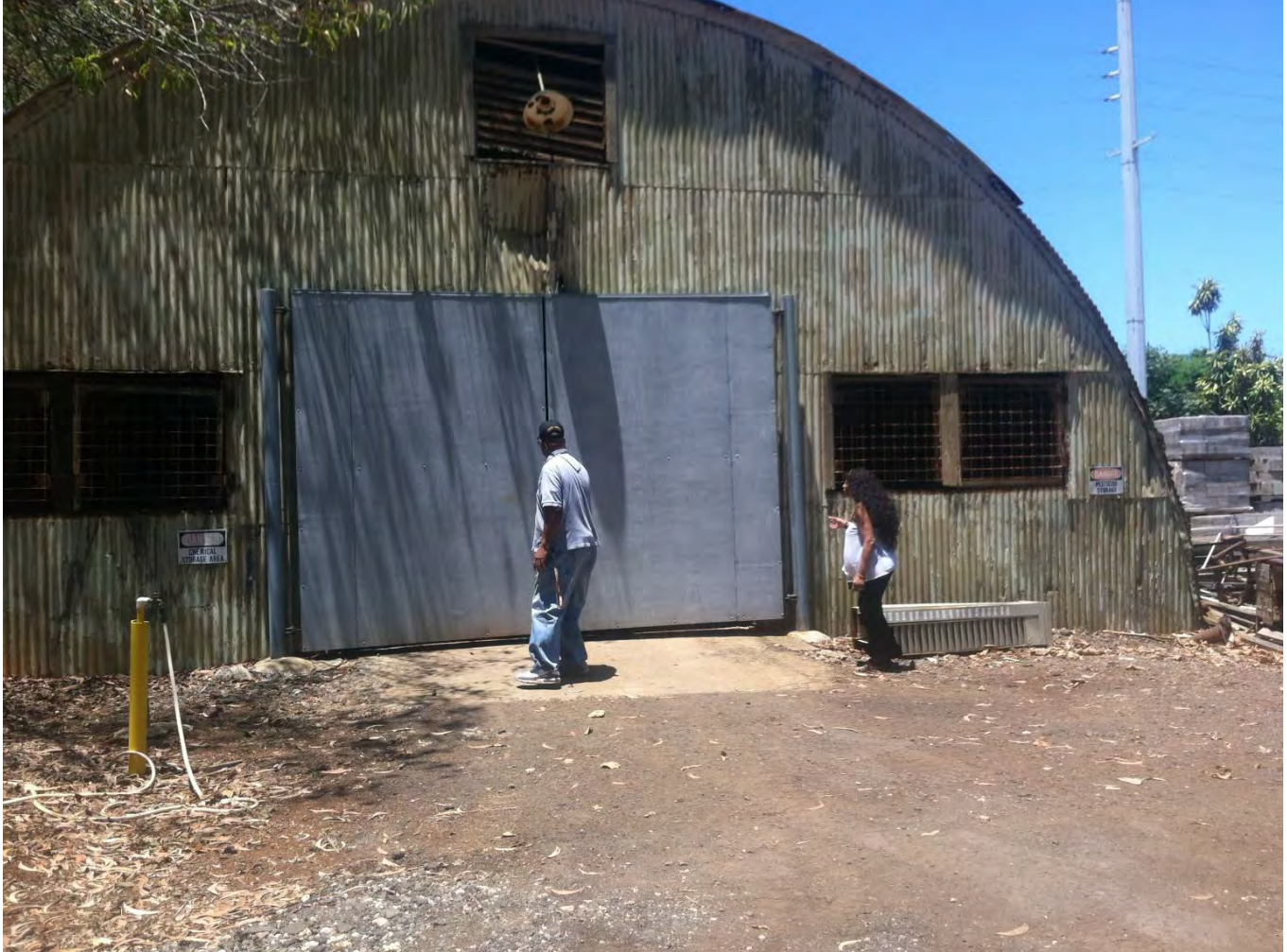
Photo 4. View of north bulkhead of Quonset Hut 33 in O’ahu Urban Garden Center, camera facing southwest. Photo by Carroll Cox. 2015.
