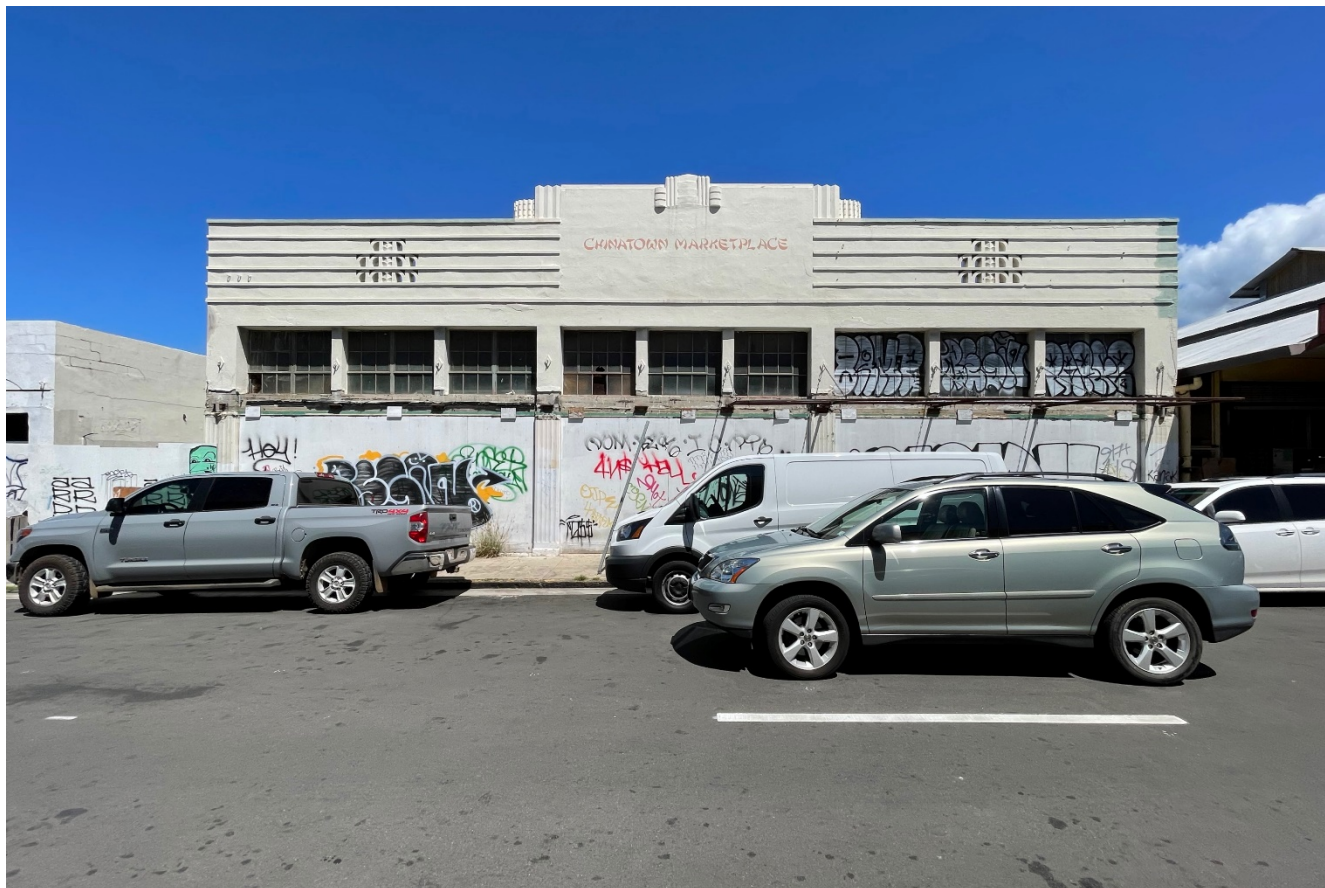
Photo Title 001 Front (southeast) facade, camera facing northwest.
