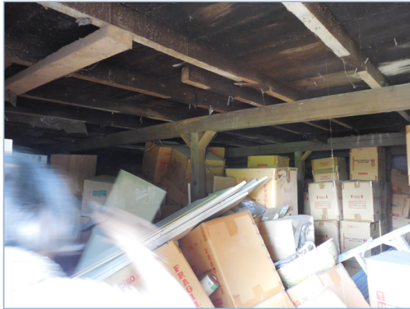
Newer understory beams supporting the older commercial story flooring.
