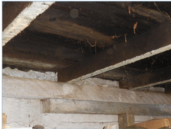
Newer understory beams supporting the older commercial story flooring.
