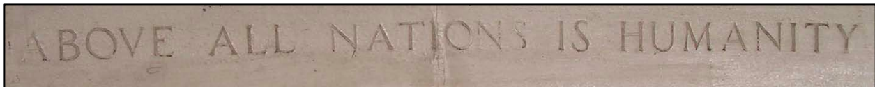
3g. Ewa engraving "Above All Nations Is Humanity" is 2.25" high and 4' 1" wide. The camera is facing NW.
