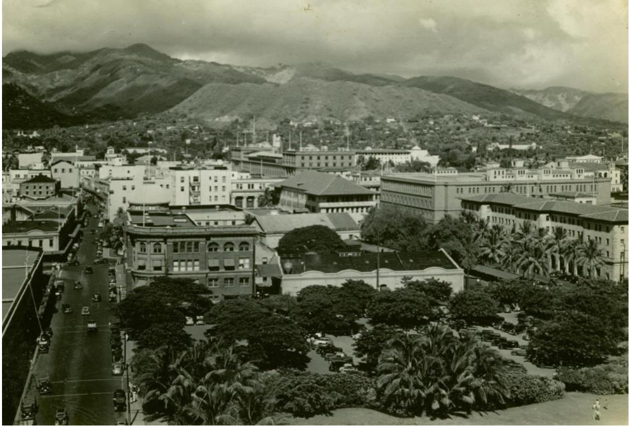
Figure 5: View of Irwin Park from atop Aloha Tower showing lush landscaping and parking, ca. 1938. (U.S. Army Museum Hawaii, No. 511)
