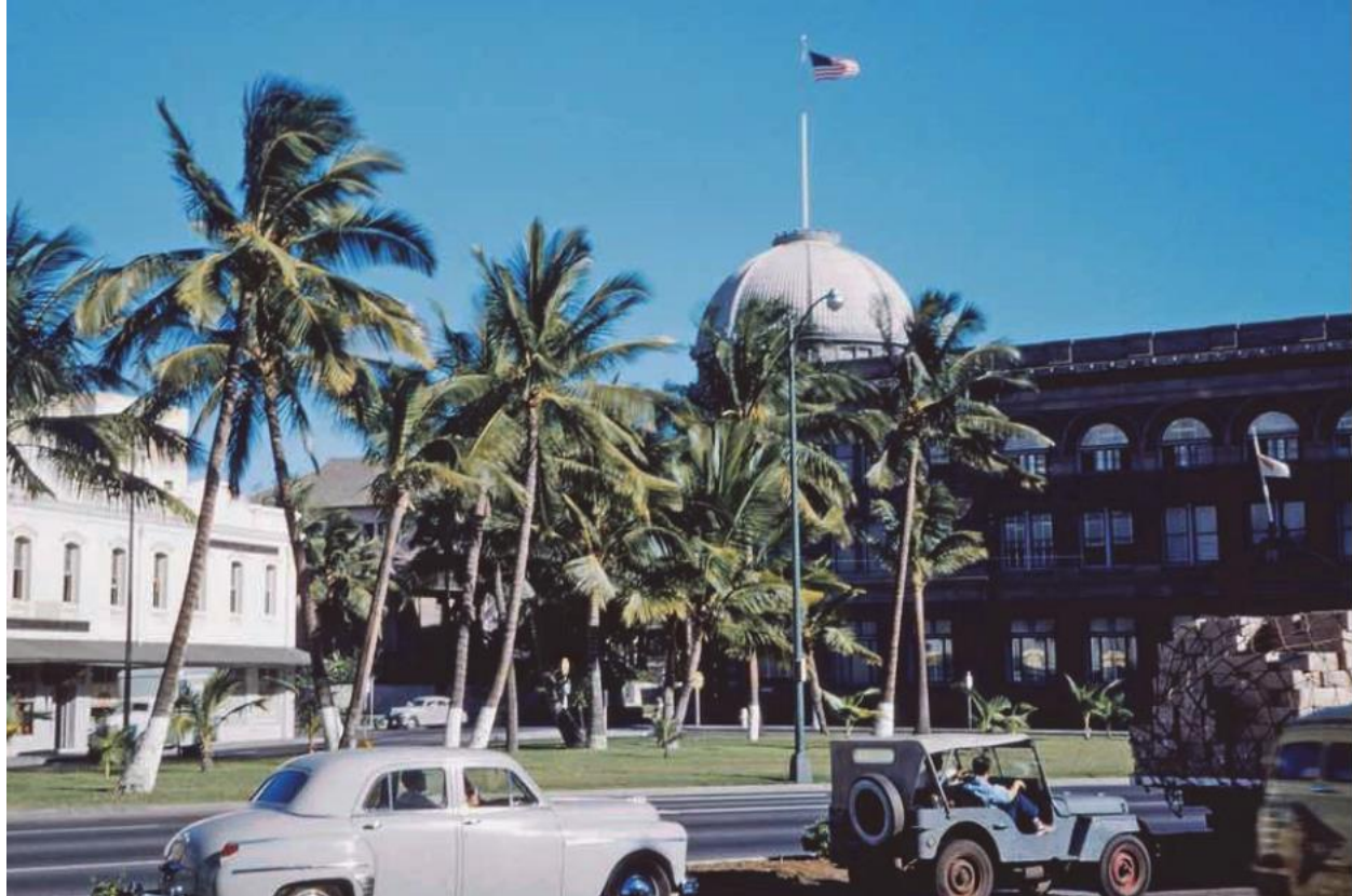
Figure 4: View of Walker Park from Nimitz Highway facing Fort Street, 1952. (Source: https://www.flickr.com/photos/kamaina56/albums/72157603803338160/page2 )
