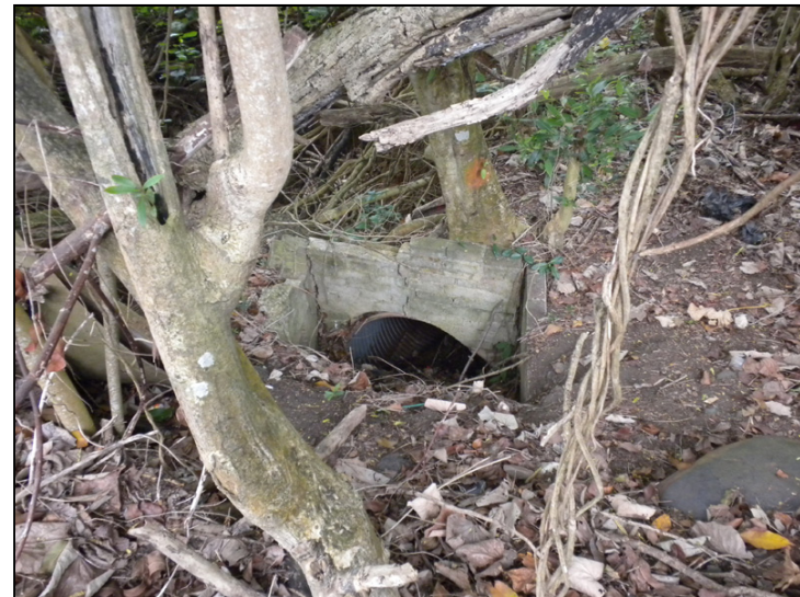
Exhibit 6 –Photo of Existing Drainage Culvert
