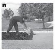
Roll out Gravelpave<sup>2</sup>, aligning the snap fit fasteners.
