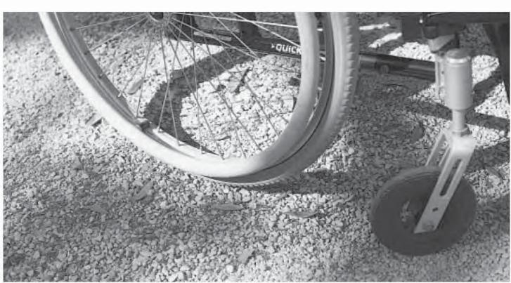
Wallace Residence, Savannah, GA—Gravelpave<sup>2</sup> creates a wheelchair-accessible surface by stabilizing gravel and supporting tire pressure. 7% dry cement was mixed with gravel before filling rings. Cover photo: Westin Kierland Resort and Spa, Scottsdale, Arizona—Grasspave<sup>2</sup> fire lane and Gravelpave<sup>2</sup> fire lane (concrete widening).
